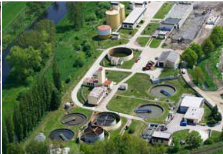
Waste-water treatment plant. © Malota / Shutterstock.com
