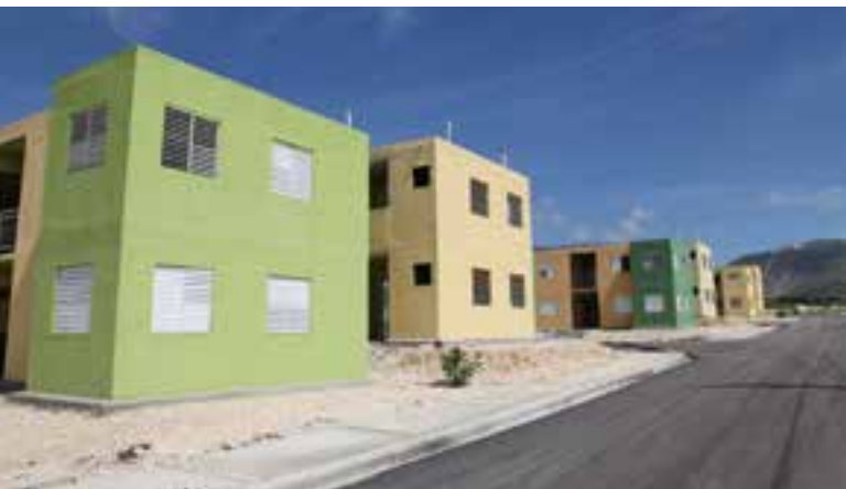
Some of the government buildings project Port-au-Prince, Haiti. © Julius Mwelu/UN-Habitat
