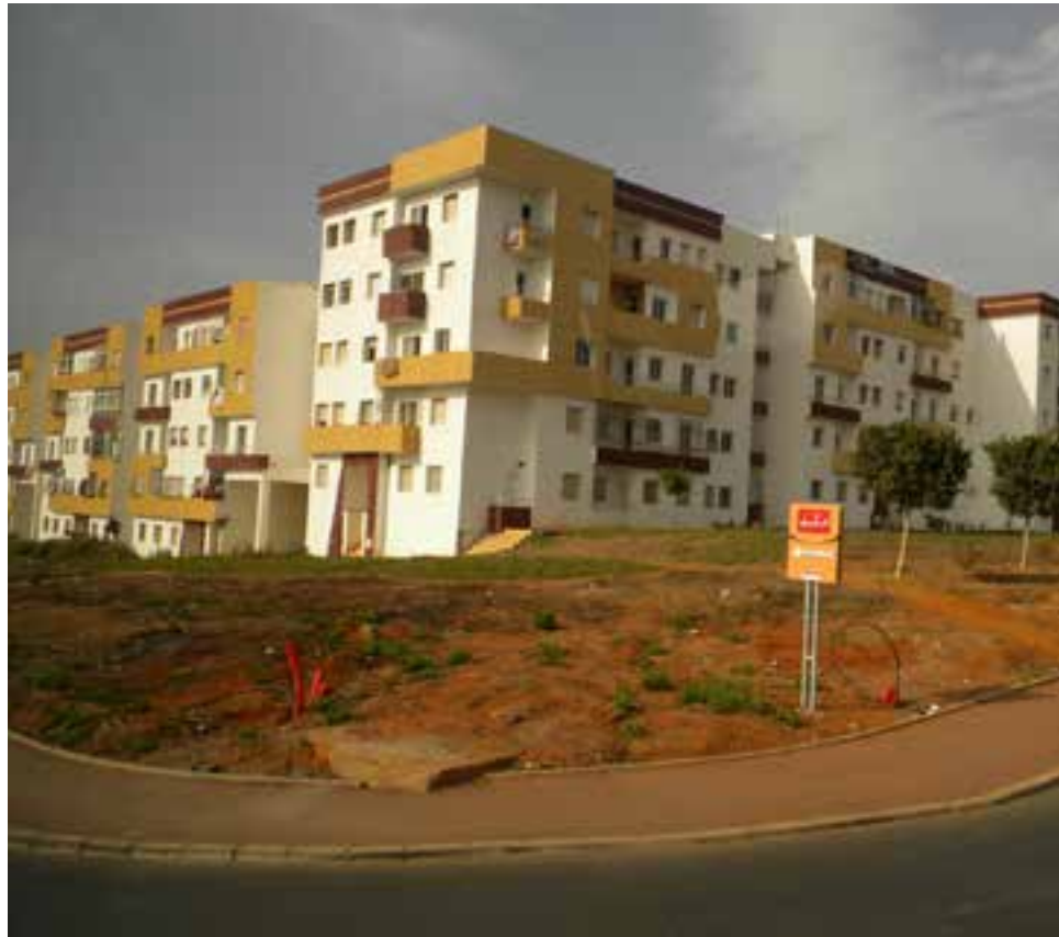
Newly constructed residential housing units in Rabat, Morocco.
