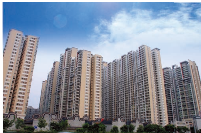
PHOTO. 10.3 Liede village after renovation Source: http://www.changye.com.cn/bbs/viewthread.php?tid=44891
