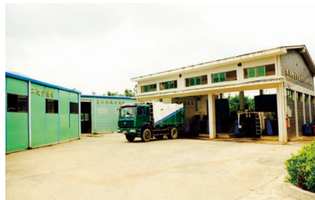
PHOTO. 8.7 Waste Transfer Station of Paitan Town Source: photographed by authors
