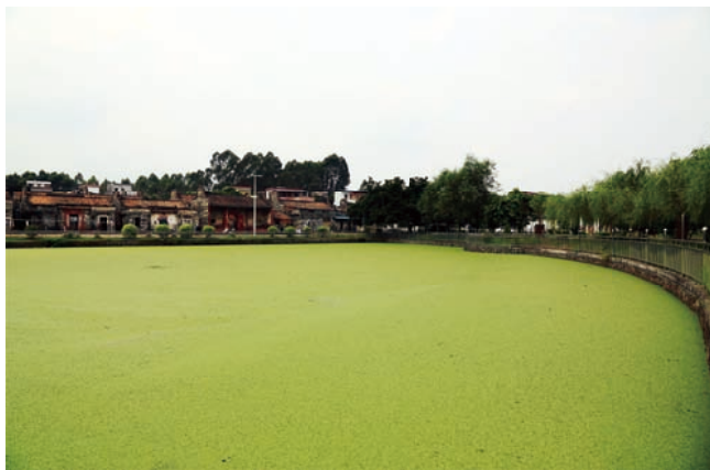
PHOTO. 8.3 Aerobic Pond Sewage Treatment Facilities Source: photographed by authors
