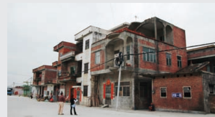
PHOTO. 14.1 Planners and villager heads reviewed the information of each renovated house
