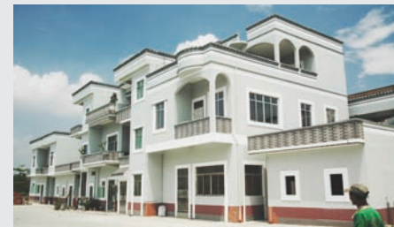
PHOTO. 14.2 the houses after renovation Source: photographed by authors
