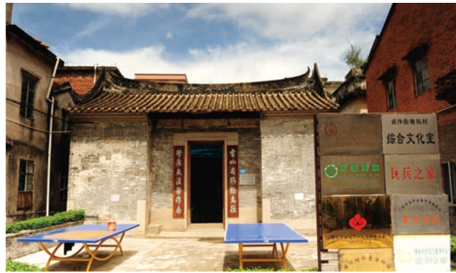
PHOTO. 11.10 Photo of the Shanxuan Study after Renovation Source: photographed by Li Xiang
