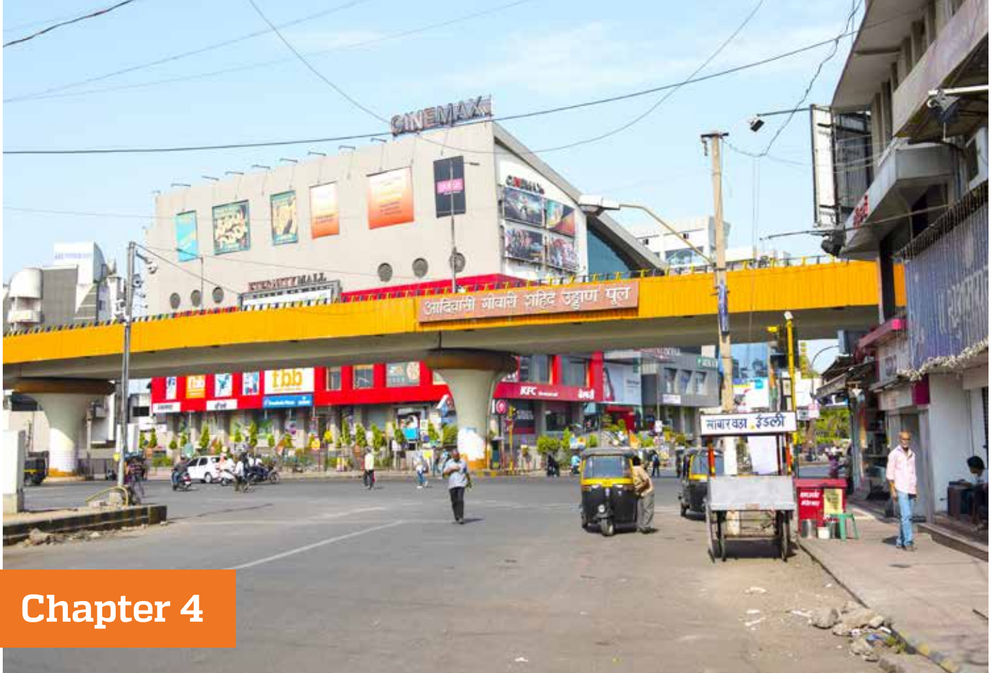
Adivasi shahid flyover bridge at Nagpur city Maharashtra India @Shutterstock
