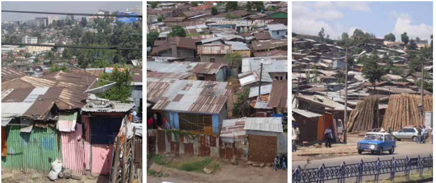
Figure 2. Conditions of the Lidata Informal Settlement before Land Readjustment
