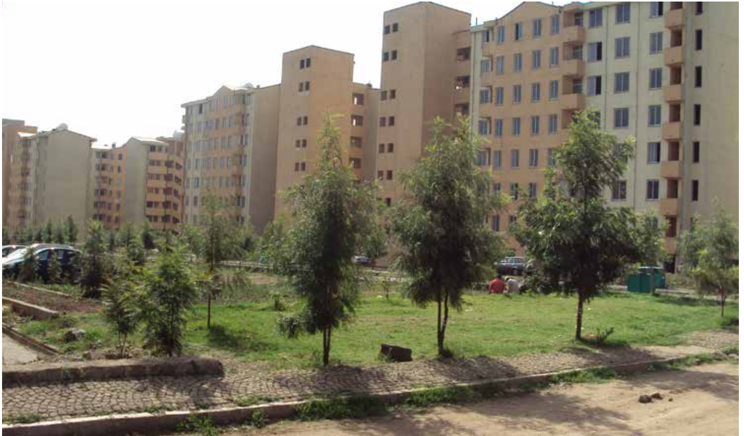
Figure 5a and b. Lidata under Construction
