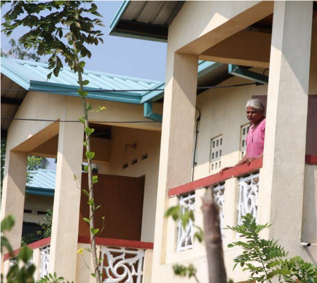
Disaster prepared construction: the 2nd Story provides a refuge against floods in Balapitiya
