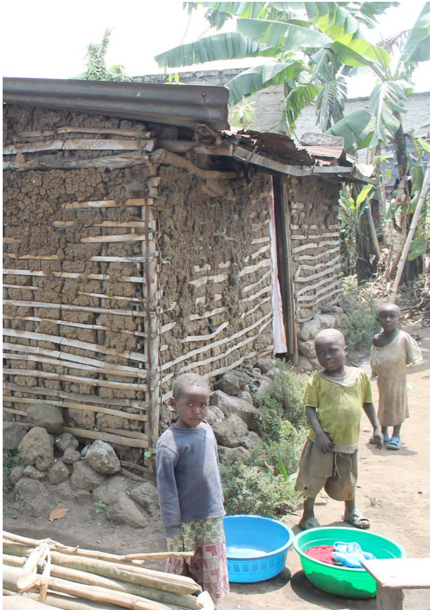
↑ Traditional wattle and daub construction. © Emma-Liisa Hannula/UN-Habitat
