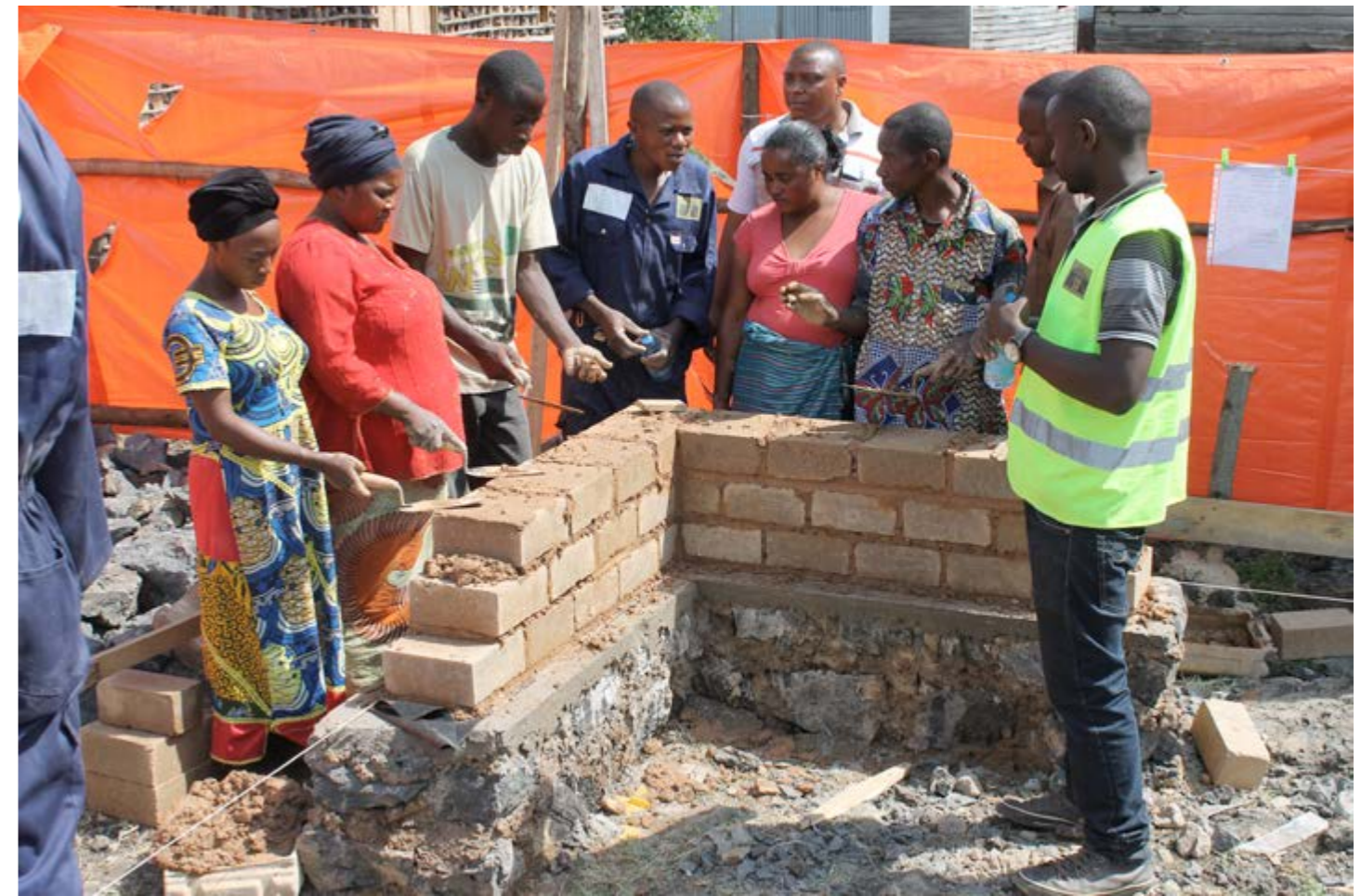
↑ Constructing the first corner of the house. © Emma-Liisa Hannula/UN-Habitat
