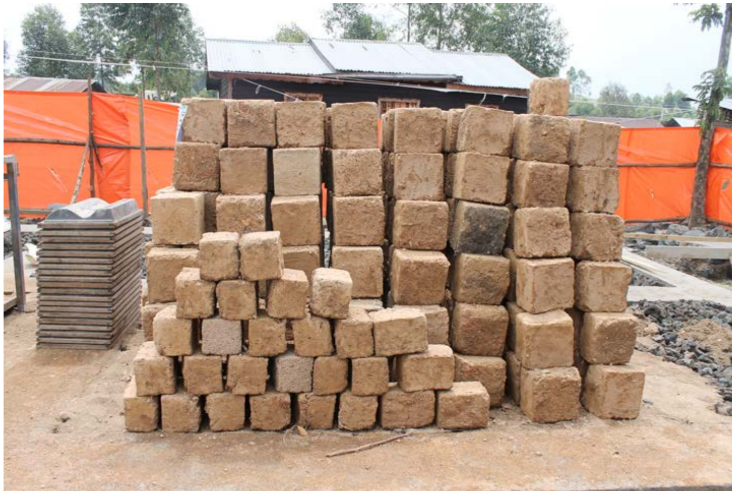
↑ Finished building blocks made from compressed earth. © Emma-Liisa Hannula/UN-Habitat
