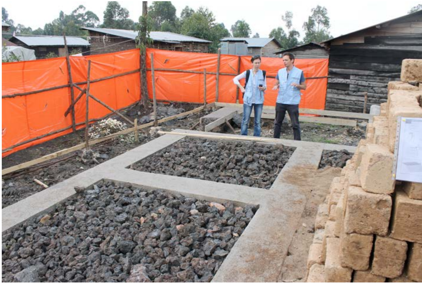
↑ Preparing the foundation. © Emma-Liisa Hannula/UN-Habitat
