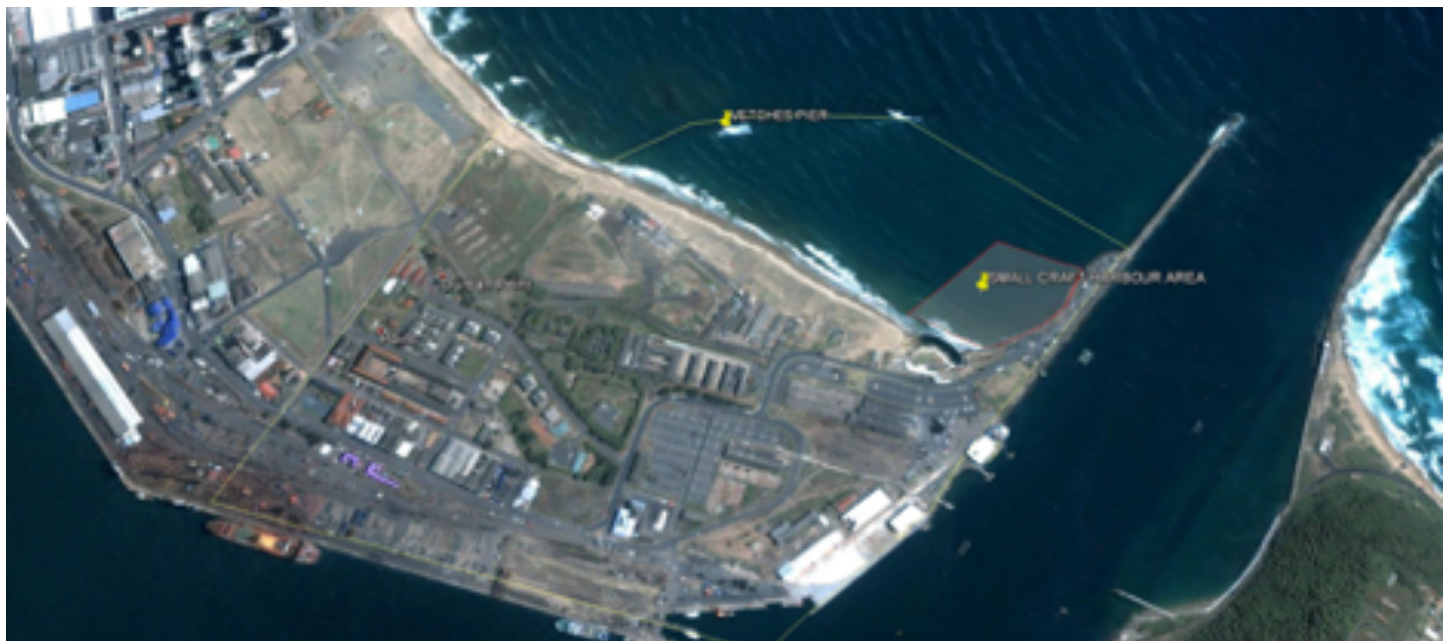
Durban Point area prior to development (2001)
