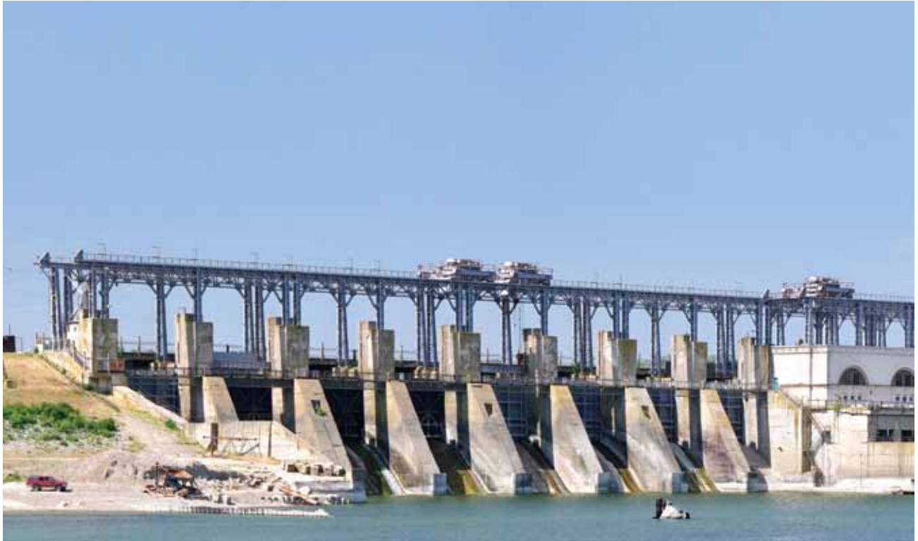
▲ The hydroelectric power station in Dubossary, Moldova. ©Serghei Starus/Shutterstock
