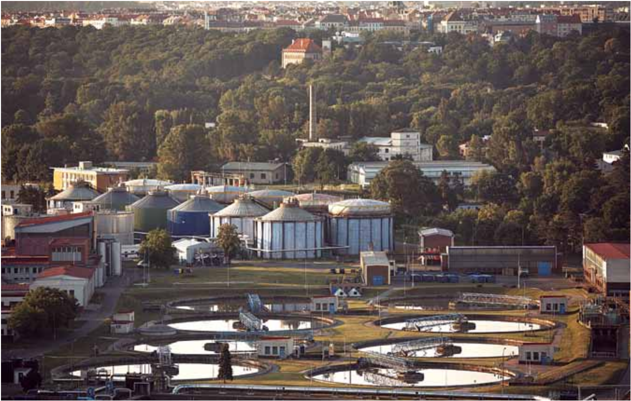
▲ A water treatment plant in Prague, Czech Republic. The Czech Republic's water supply and wastewater treatment services are highly privatised. ©Chalabala/Shutterstock
