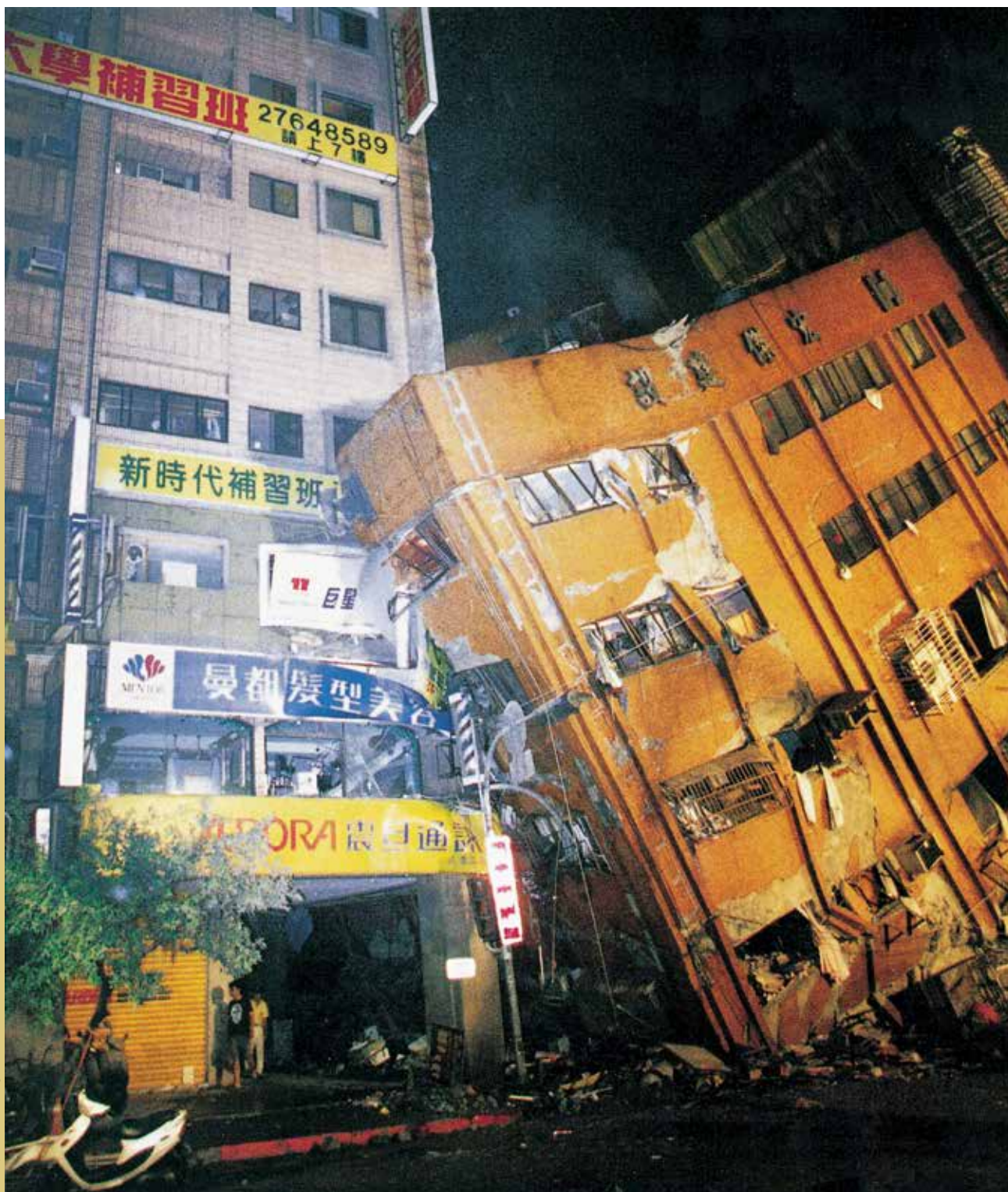
中国台湾省一幢在地震后倒塌的建筑 Collapsed buildings after an earthquake in the Taiwan Province of China LO TSUNG HSIEN/UNEP/STILL PICTURES
