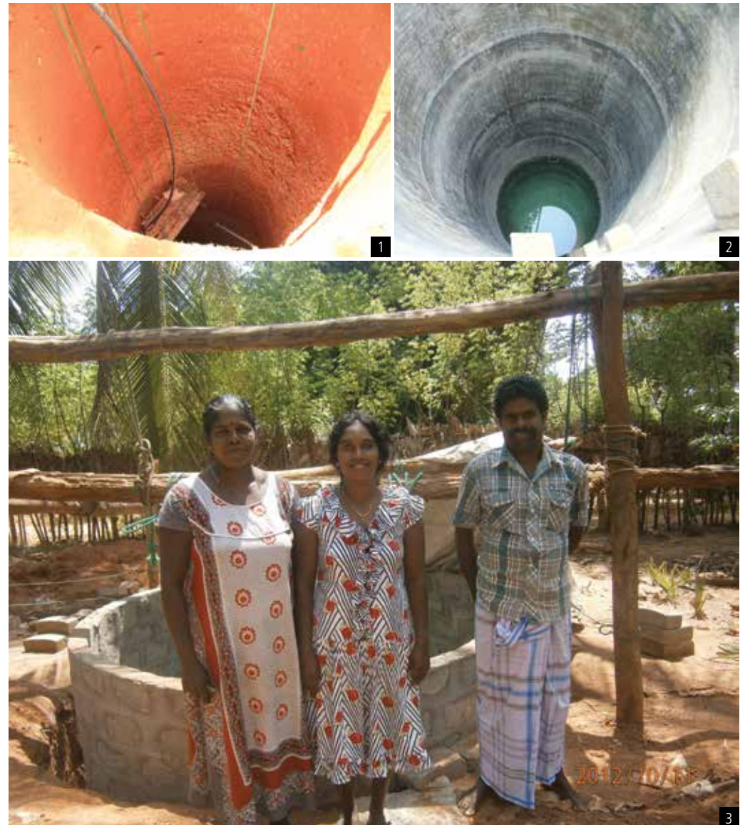
1, 2 & 3: Construction of community well in Mamoolai village, Mullaitivu.
