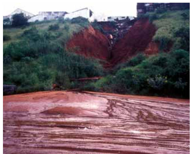
Soil erosion on Avendia OUA in Maputo, Mozambique.
