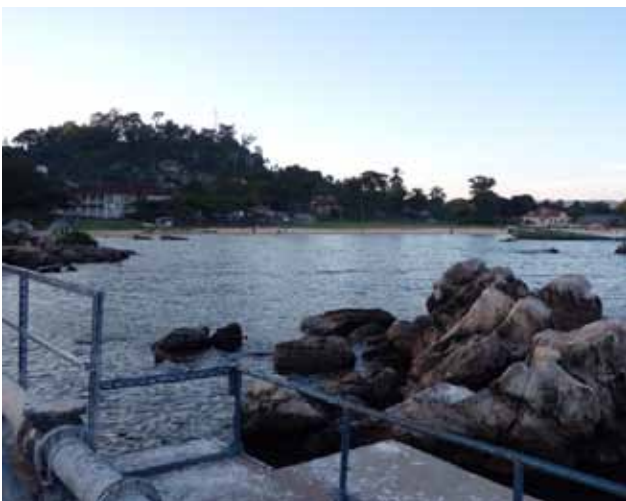
Intake for water supply system in Bukoba, Tanzania.
