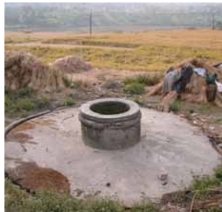
FIGURE 3.4 Biogas Connection and Improved Traditional Well Khokhana, Lalitpur
