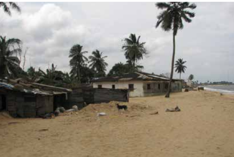
Figure 52. New Kru Town houses on the beach and inundated by sand after high tide on 7th August, 2013
