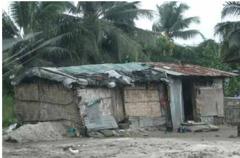
Figure 25. Very poor housing, using bamboo mats, metal sheeting and poles, on the periphery of Monrovia
