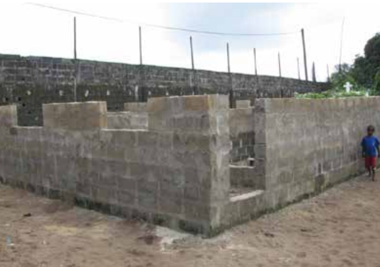
Figure 80. A house in New Kru Town undergoing incremental development, completed up to sill level
