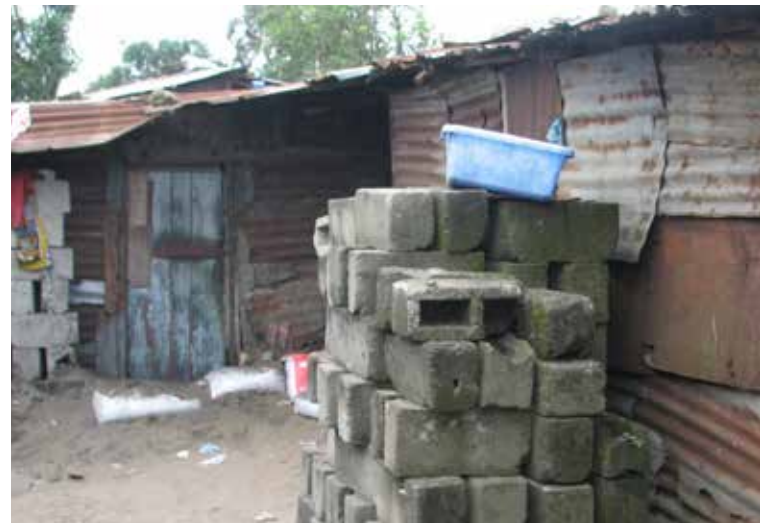
Figure 78. Block saving in New Kru Town against the time when the wood and metal sheet structure can be upgraded to cement blocks
