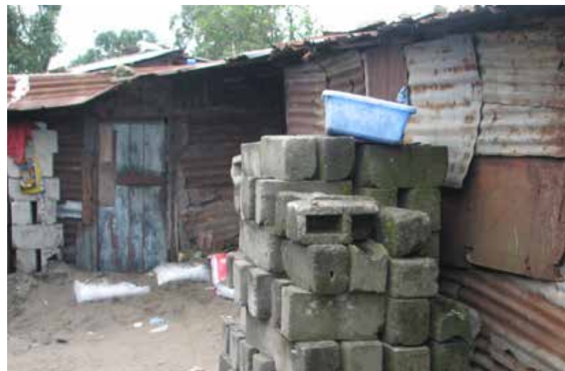
Figure 82. Multi-storey slab and frame structure being built in Monrovia
