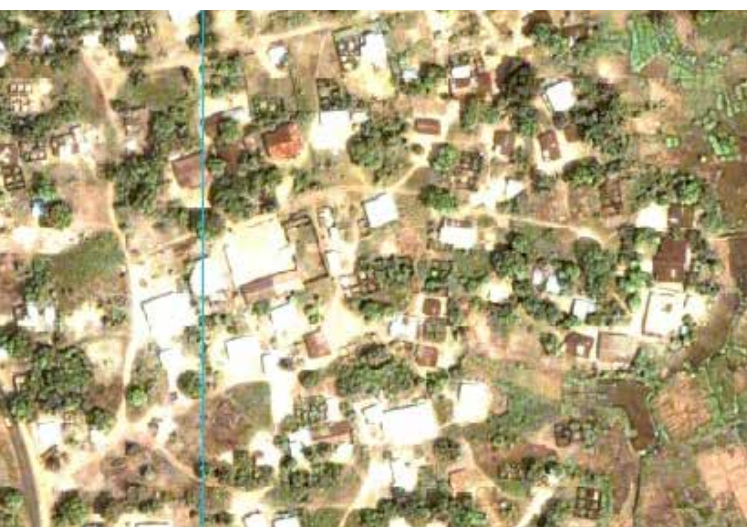
Figure 81. Peripheral development in Monrovia with many unfinished houses
