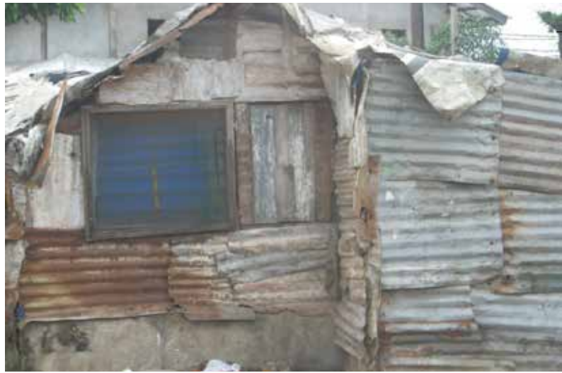
Figure 24. Poor quality housing in wood poles and metal sheets, New Kru Town
