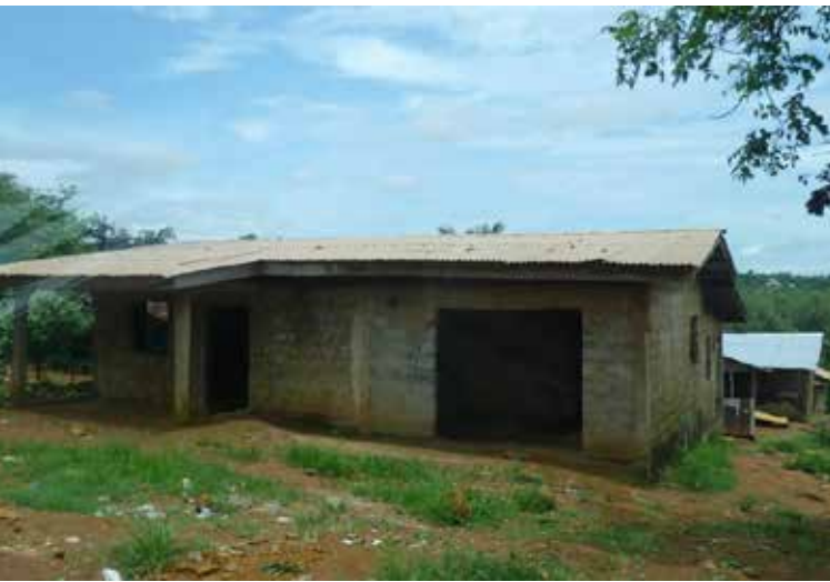
Figure 79. Houses like this in Peace Island can be built for as little as $5,000
