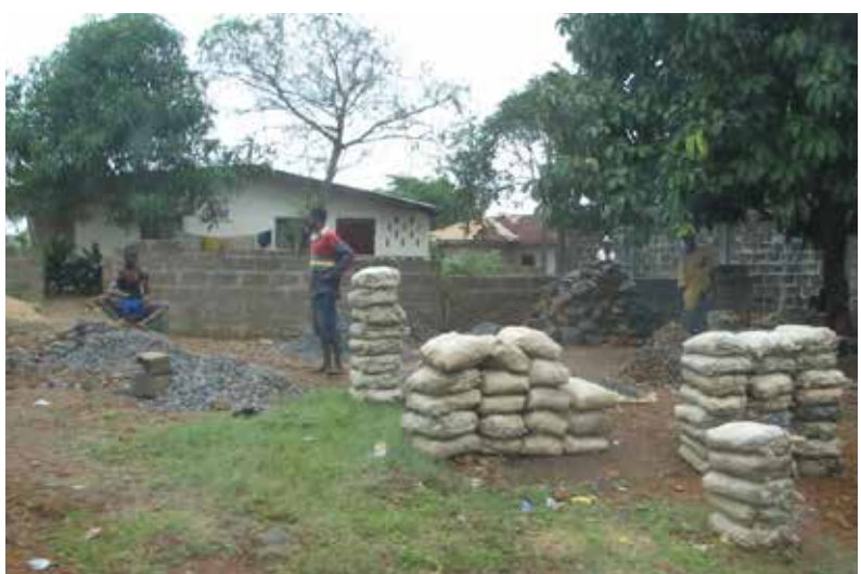
Figure 85. Aggregate crushing by hand (left) and for sale by the bag, Monrovia
