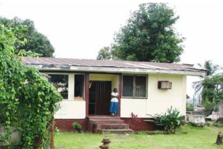
Figure 7. NHA housing in New Matadi
