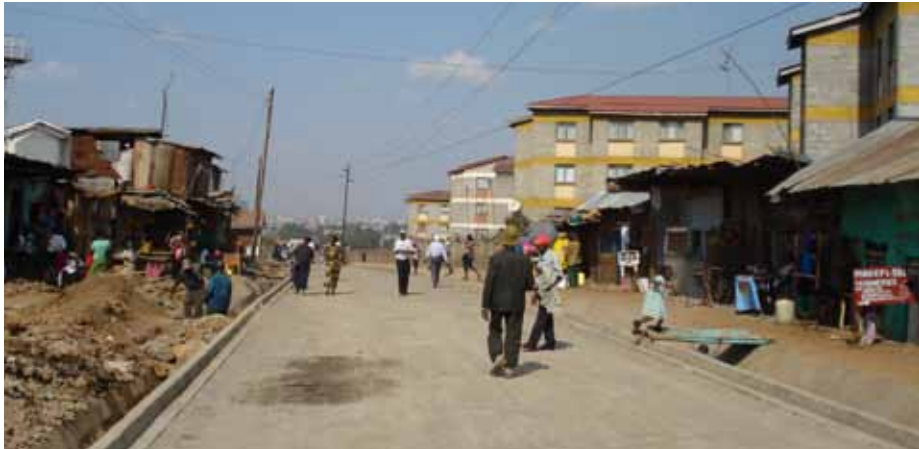
FIGURE 3.1: New 12m road Kibera - labour based construction
