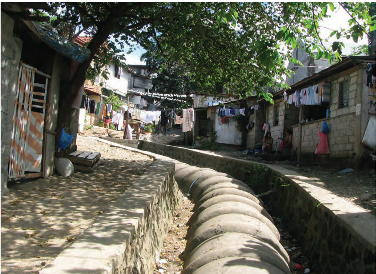
Example of site improvement required by the housing project: a permanent riprap in Payatas
