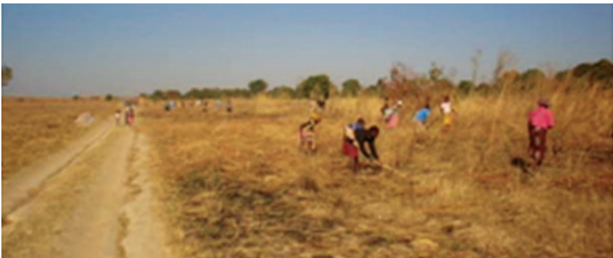
Preparing road clearances. © Development Workshop
