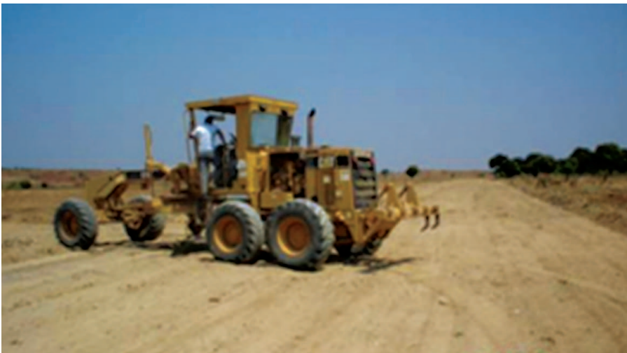
Preparing road clearances. © Development Workshop
