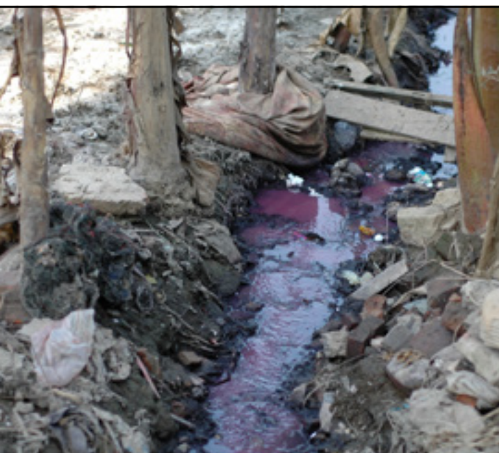
Figure 27: Open drainage in Van Phuc silk village, Ha Dong, Hanoi
