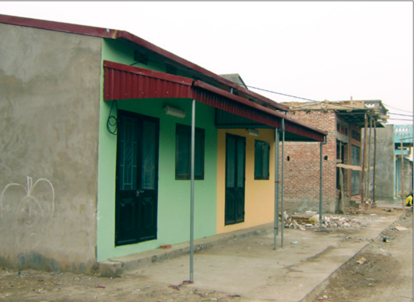
Figure 8: Resettlement houses in Hai Duong built by Habitat for Humanity Source: 2010 © UN-Habitat/ Nguy Ha
