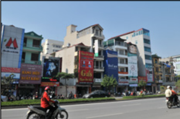
Figure 10: Type A permanent - Modern shop houses in Hanoi
