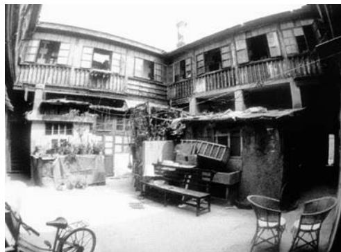
Figure 3.19 Residential Buildings at Binhai Jingqu before Upgrading
