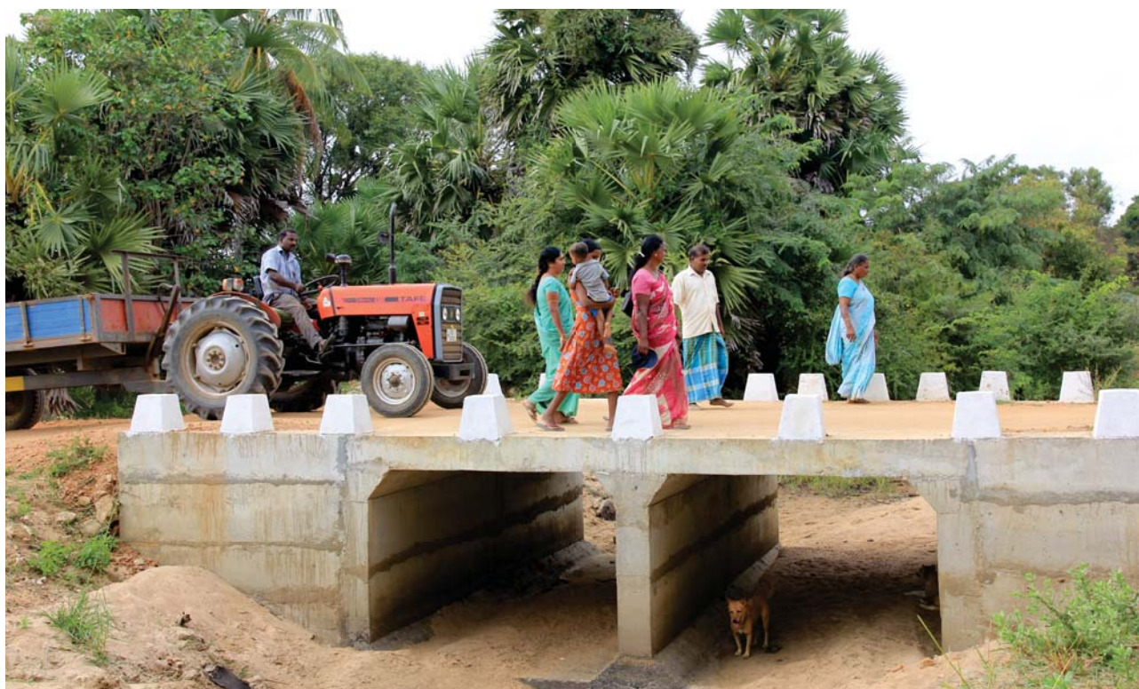
The storm water drainage system constructed in Puliampokkanai GN division.
