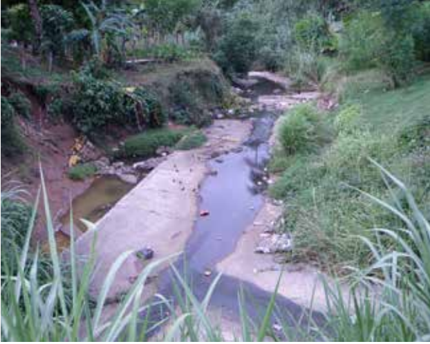
Poor drainage systems in Lautoka © SCOPE
