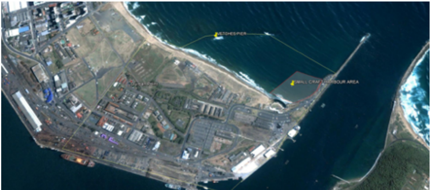
Durban Point area prior to development (2001)
