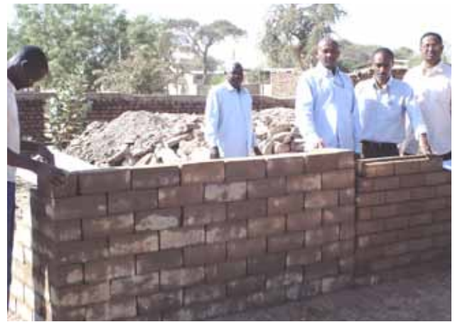
Building with alternative technologies
