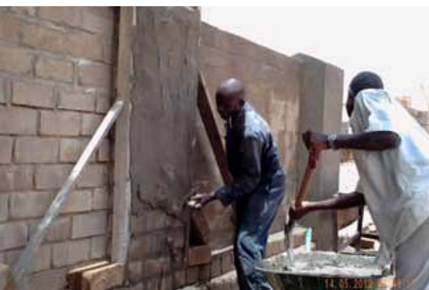
Examples of plastering and finishing
