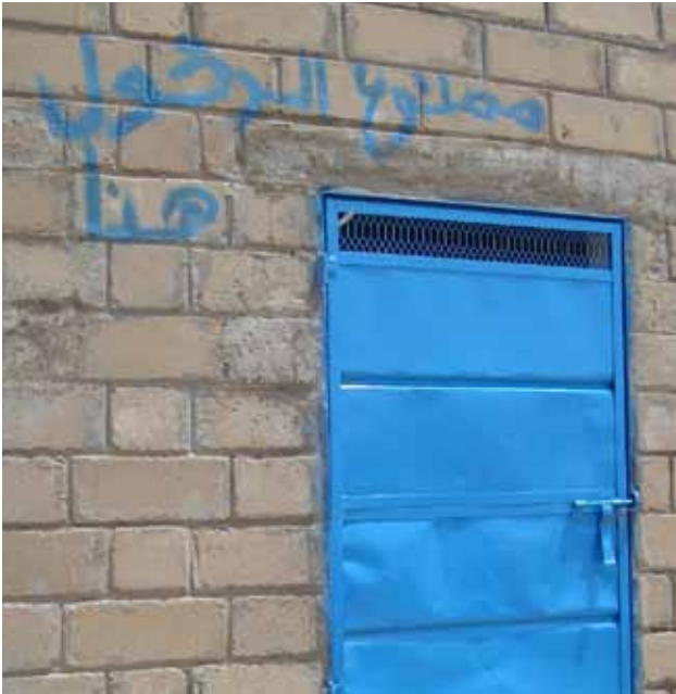
Public latrine in Nyala
