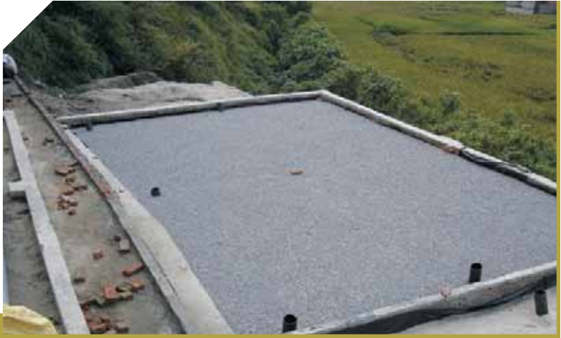
Filling of substrate completed in vertical flow CW
