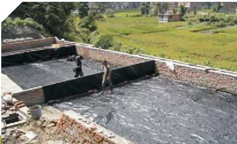
Plastic liners placed in the basin
