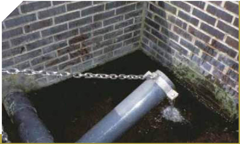
Swivelling elbow outlet (Cooper et al. , 1996)
