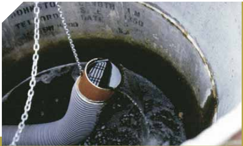
Flexible pipe outlet (Cooper et al. , 1996)
