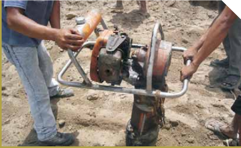
Compaction of the subgrade works
