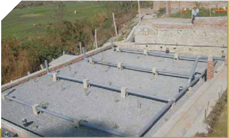
Vertical flow CW after laying of inlet distribution network and plantation of vegetation
