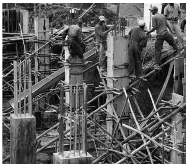
Figure 31: Labourers building the foundations for Lideta condominiums Lideta, Addis Ababa.
