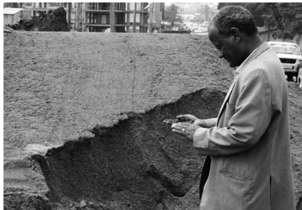
Figure 27: Quality checks on building materials are crucial to ensure a high-quality result. Lideta, Addis Ababa. © UN-HABITAT/ Katherine Hegab
