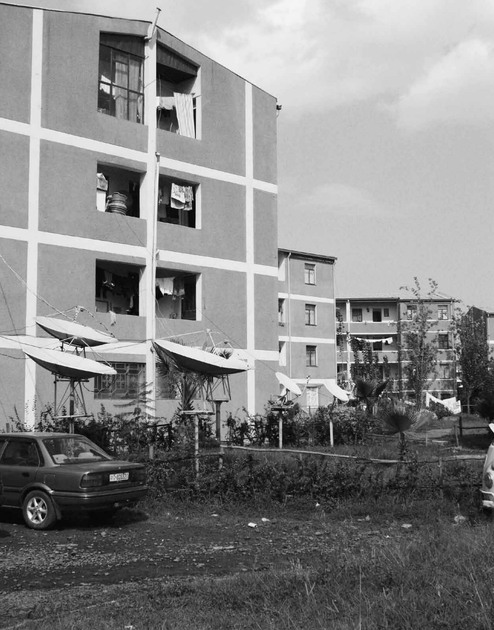
Figure 1: The Pilot Project for the Condominium Housing Programme built in Bole Gerji. Bole Gerji, Addis Ababa. © UN-HABITAT / Katherine Hegab
