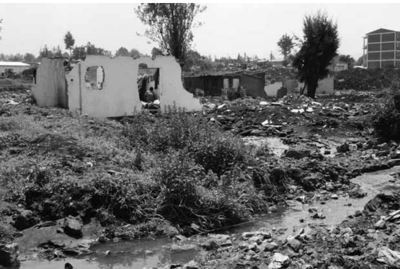
Figure 25: Lideta site being cleared. © UN-HABITAT/ Katherine Hegab
