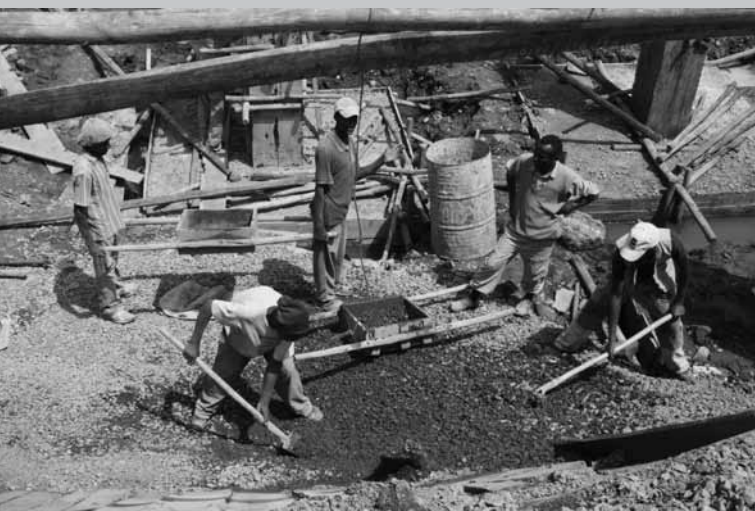
Figure 10: Construction methods in Ethiopia are labour intensive. © UN-HABITAT
