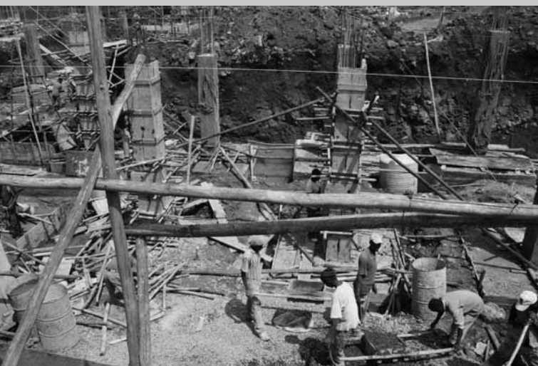
Figure 11: Multi-storey buildings in Addis Ababa are typically constructed from cast in-situ reinforced concrete frame with brick infill walls. © UN-HABITAT
