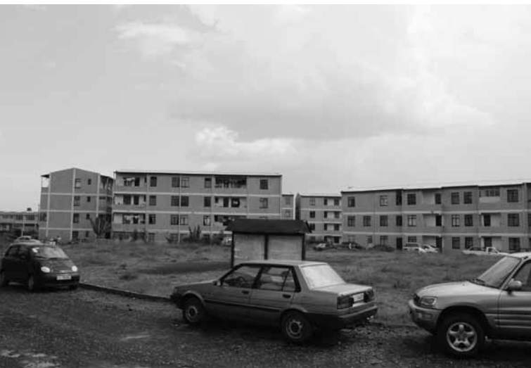
Figure 12: Condominium housing of the Integrated Housing Development Programme. © UN-HABITAT
