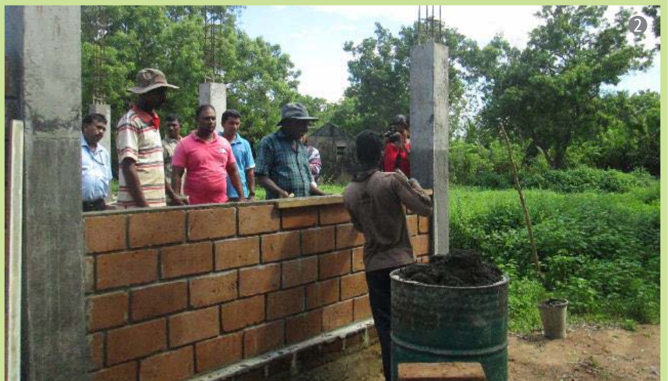
Mahilavedduwan Community Centre walls being constructed using mud concrete blocks.
