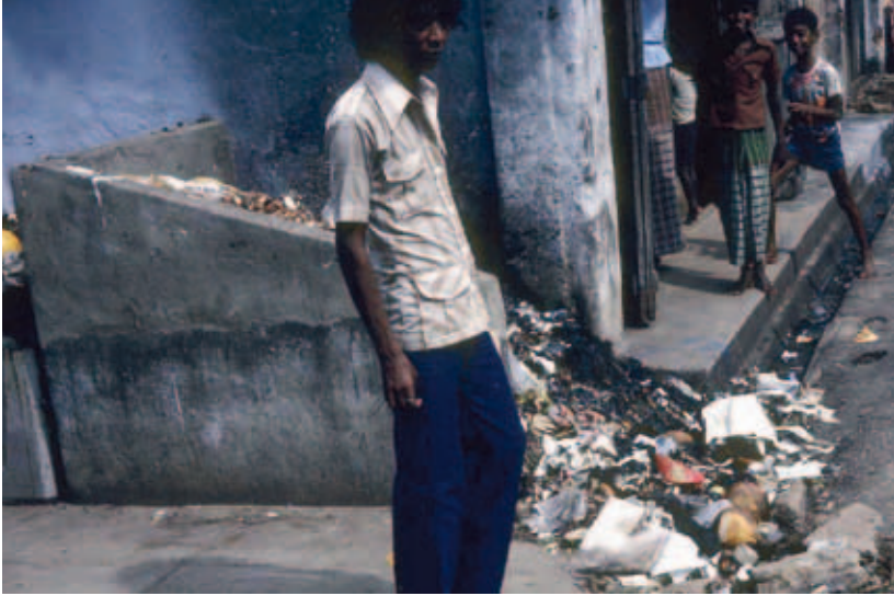
Waste containers should not be located next to open drains. Here, waste from the bunker is blocking the drain.
