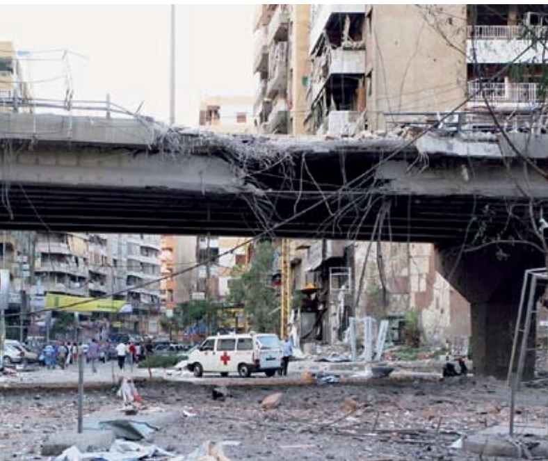
Bir el-Abed, southern Beirut, damaged by an Israel air strike 16 July 2006. Photo © L. Hatoum/IRIN
