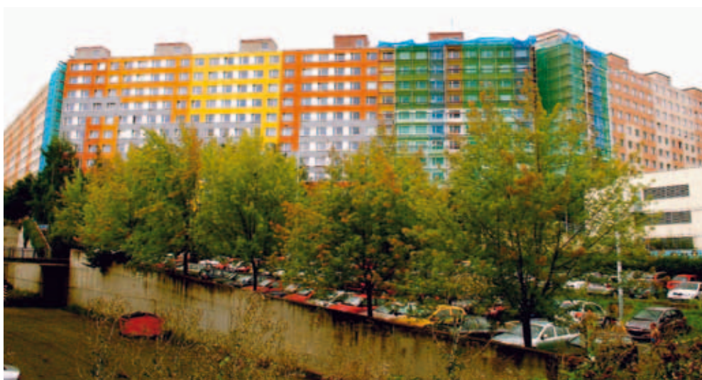
Figure 35: Housing undergoing rehabilitation as part of the Czech Republic upgrading programme.
