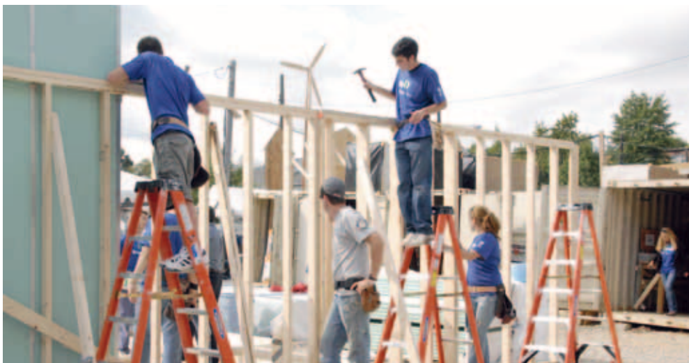
Figure 17: New housing construction in the United States. Photo © UN-HABITAT
