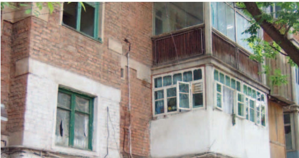
Figure 21: Occupant additions and modifications to multi-household housing in Tajikistan Photo © UN-HABITAT/Claudio Acioly
