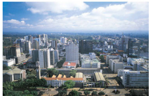
Plate 5,6 & 7: Above: Aerial view of a Maasai Homestead; Middle: the settlement grid of Nairobi CBD; Below: Nairobi's skyline. Source: Internet Sources
