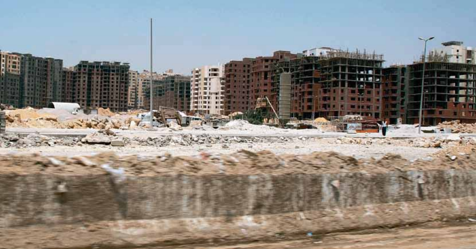
Blocks of empty and/or unfinished apartments around the Cairo ring road.
