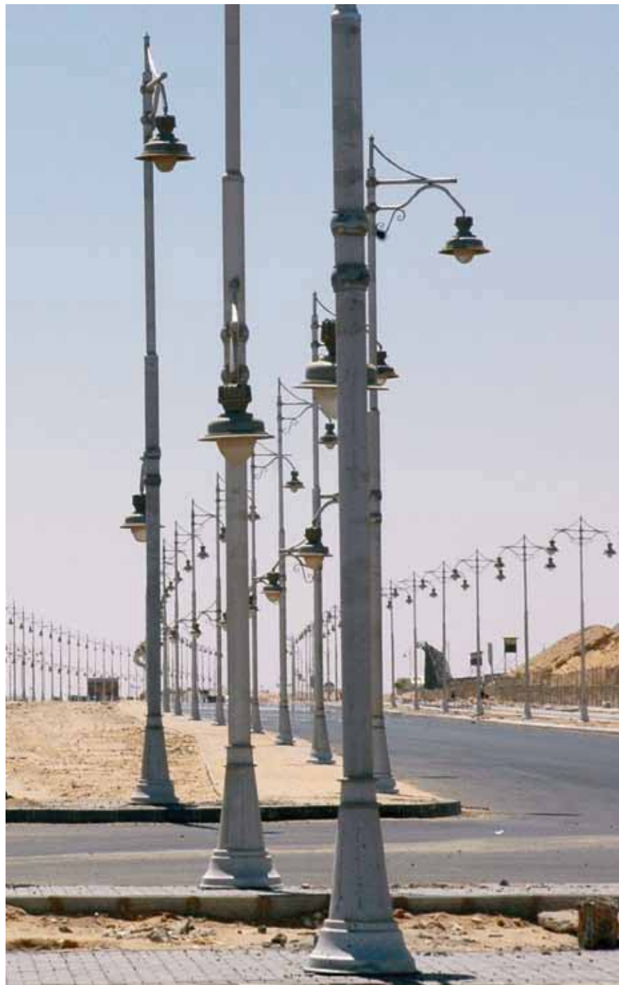
Infrastructure of well-constructed roads and extensive street-lighting prepare the way for development into the desert. New Cairo
