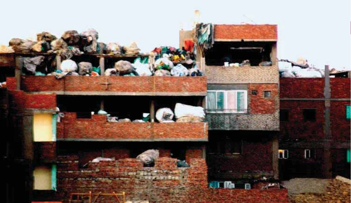
Rubbish stored on roofs in the informal settlement dominated by the Zabbaleen, in the sprawling Manshiet Nassr settlement.
