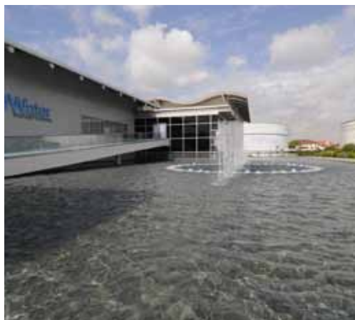
NEWater Visitor Centre, Koh Sek Lim Road, Singapore © PUB, Singapore's national water agency, 2009
