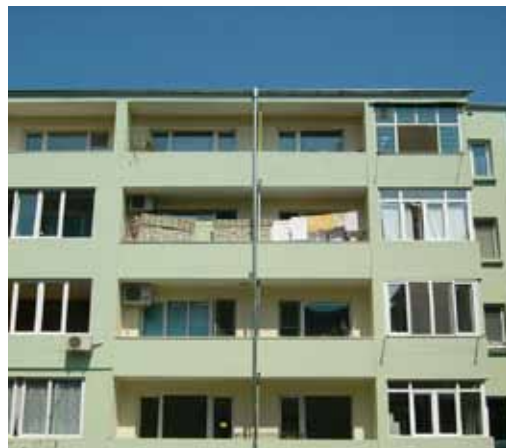
Apartments at 6 Saglasie Str., bl. Poshtenez 2, Burgas - after renovation
