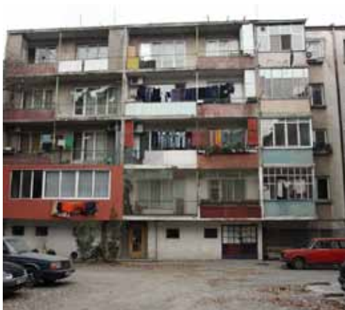
Apartments at 6 Saglasie Str., bl. Poshtenez 2, Burgas - before renovation
