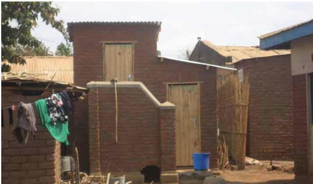
Front view of the ecosan toilet (raised structure on left) and adjoining shower (ground level on right). The ecosan toilet is raised above two composting chambers with access to the chambers at the rear of the structure © Lauren Tavener-Smith, September 2011
