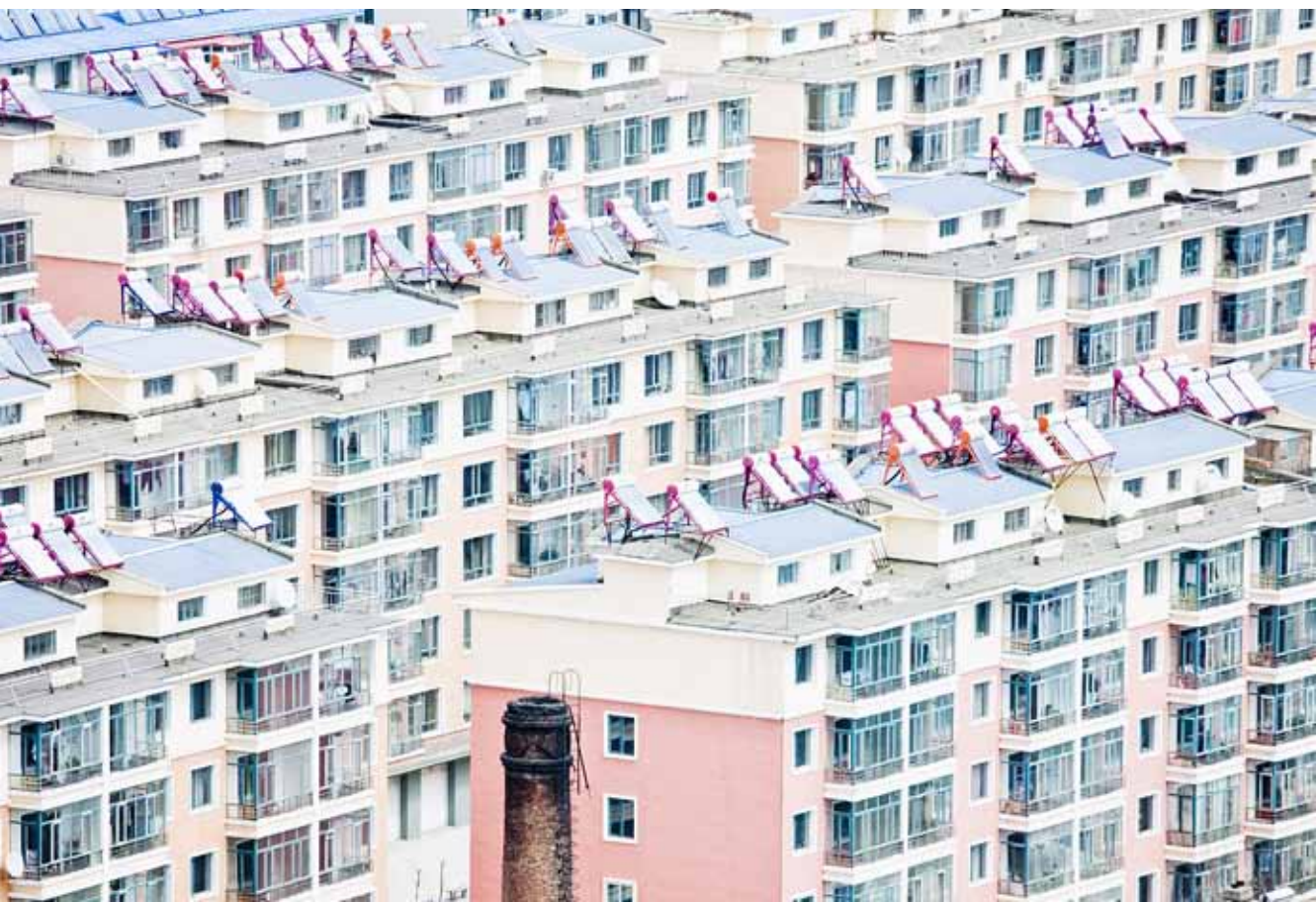
Solar hot water heaters on newly built apartment blocks in Hunchun, China © UN-Habitat/Alessandro Scotti
