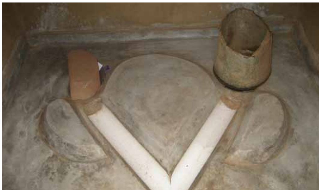
Inside the ecosan squat toilet, urine is diverted through a hole at the apex of the v-shaped gutter where it is soaked away or collected in jerry cans. The brick and bucket cover two holes for faeces, above two chambers. At any one time, one hole and chamber is in use, whilst the contents in the other chamber decompose © Lauren Tavener-Smith, September 2011
