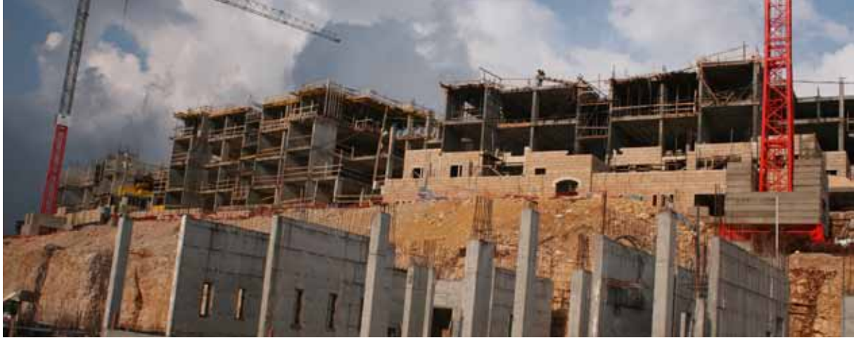
A construction site in Ramallah, Occupied Palestinian Territory © UN-Habitat
