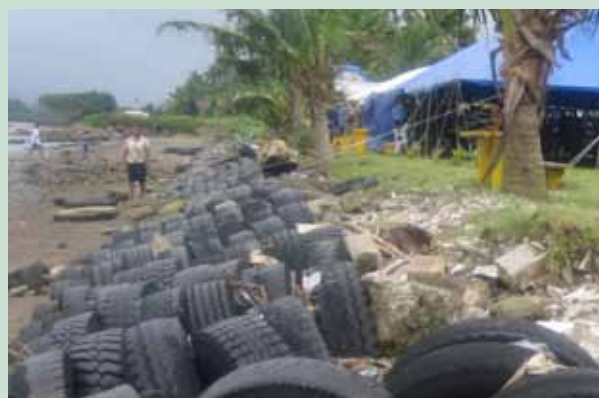
Coastal protection structures in Lami, Fiji © UN-Habitat
