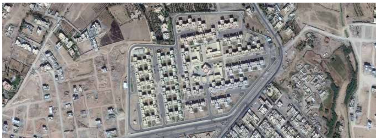
Al-Hadba Housing Project, north of Mosul © DigitalGlobe, 16 October 2016 Source: US Department of State, NextView License
