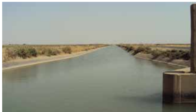
Al-Jazira irrigation project © UN-Habitat / Iraqi Urban Observatory
