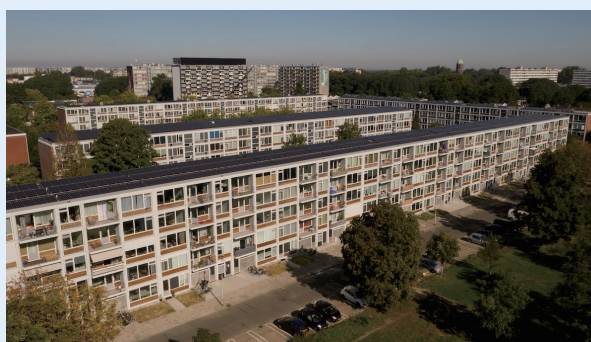
Figure 9.1 A completed Energiesprong net-zero retrofit renovation of an outdated Intervam apartment complex in Utrecht, the Kingdom of the Netherlands
