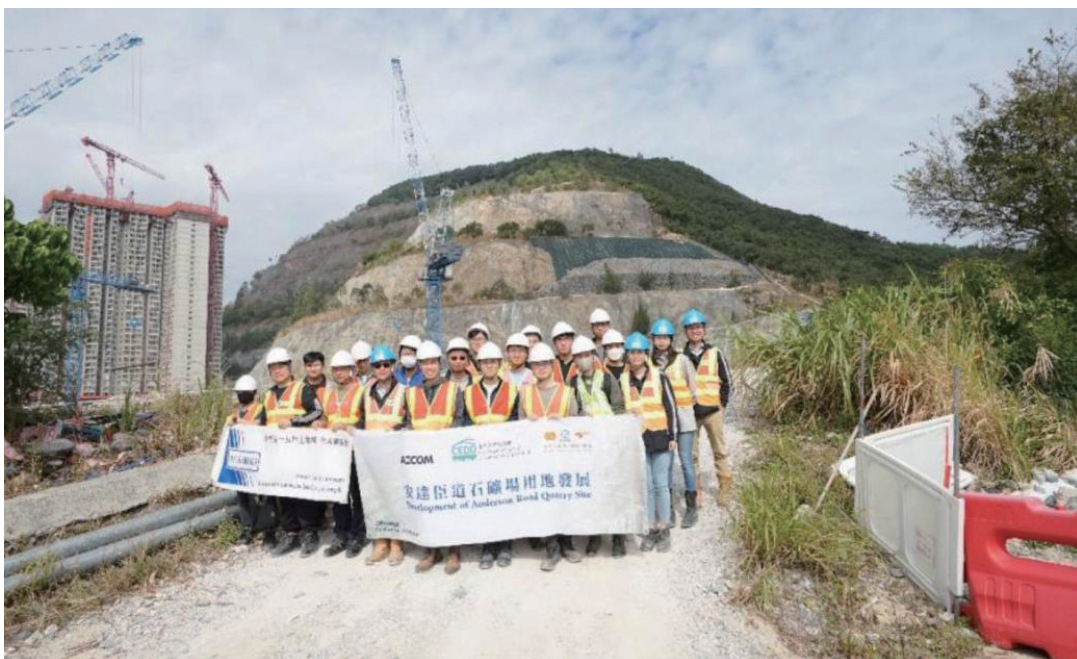
Source: Provided by Civil Engineering and Development Department, the Government of the Hong Kong Special Administrative Region Figure 6.7 Professional organizations visit the construction site
