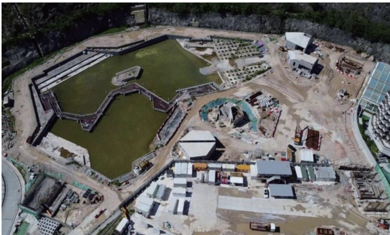
Figure 6.5 The artificial stormwater storage lake under construction
