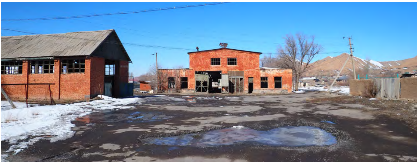
Figure 7. Existing condition of the industrial site
