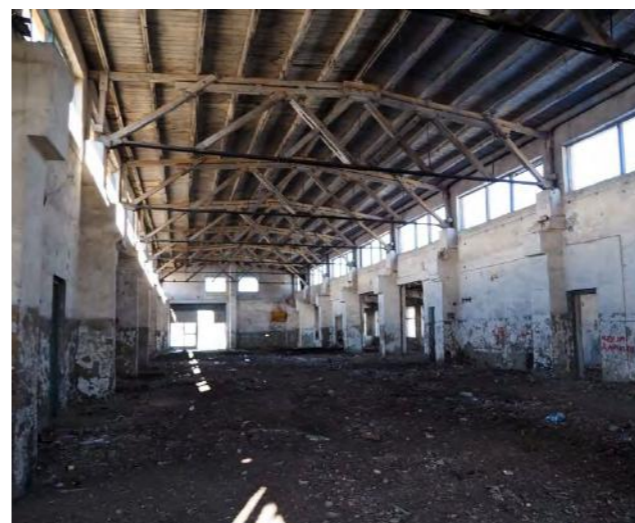
Figure 8. Existing condition of the warehouse
