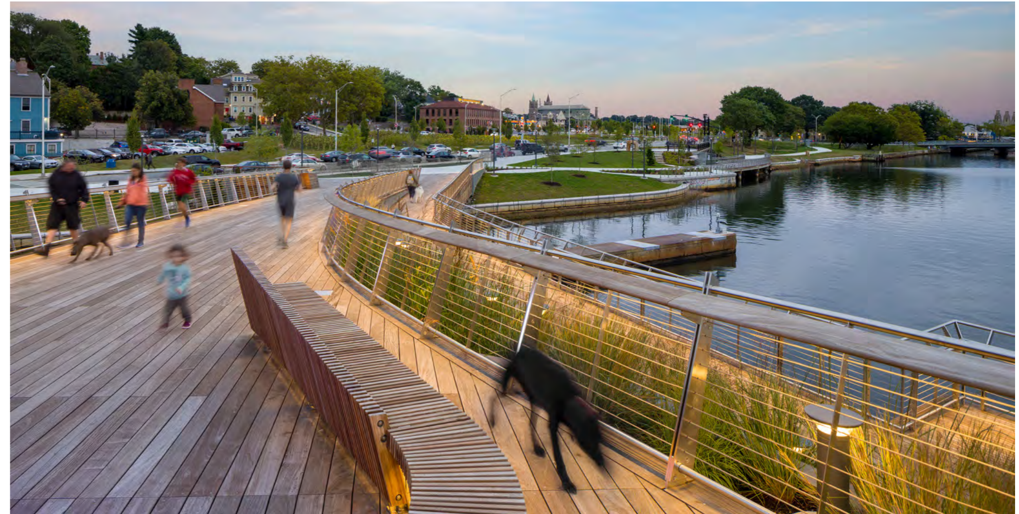
Figure 35. Integration of urban furniture in bridge design Source: Steve Kroodsma, design by Inform Studio + Büro Happold
