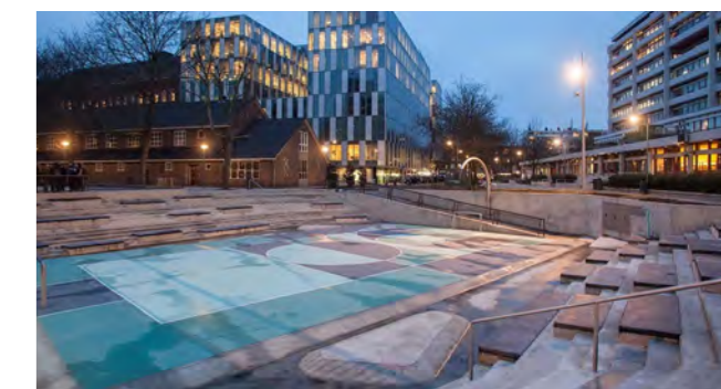
Figure 36. Water Square* in Bentheimplein. Example of public space design that integrates stormwater retention. Source: www.publicspace.org
