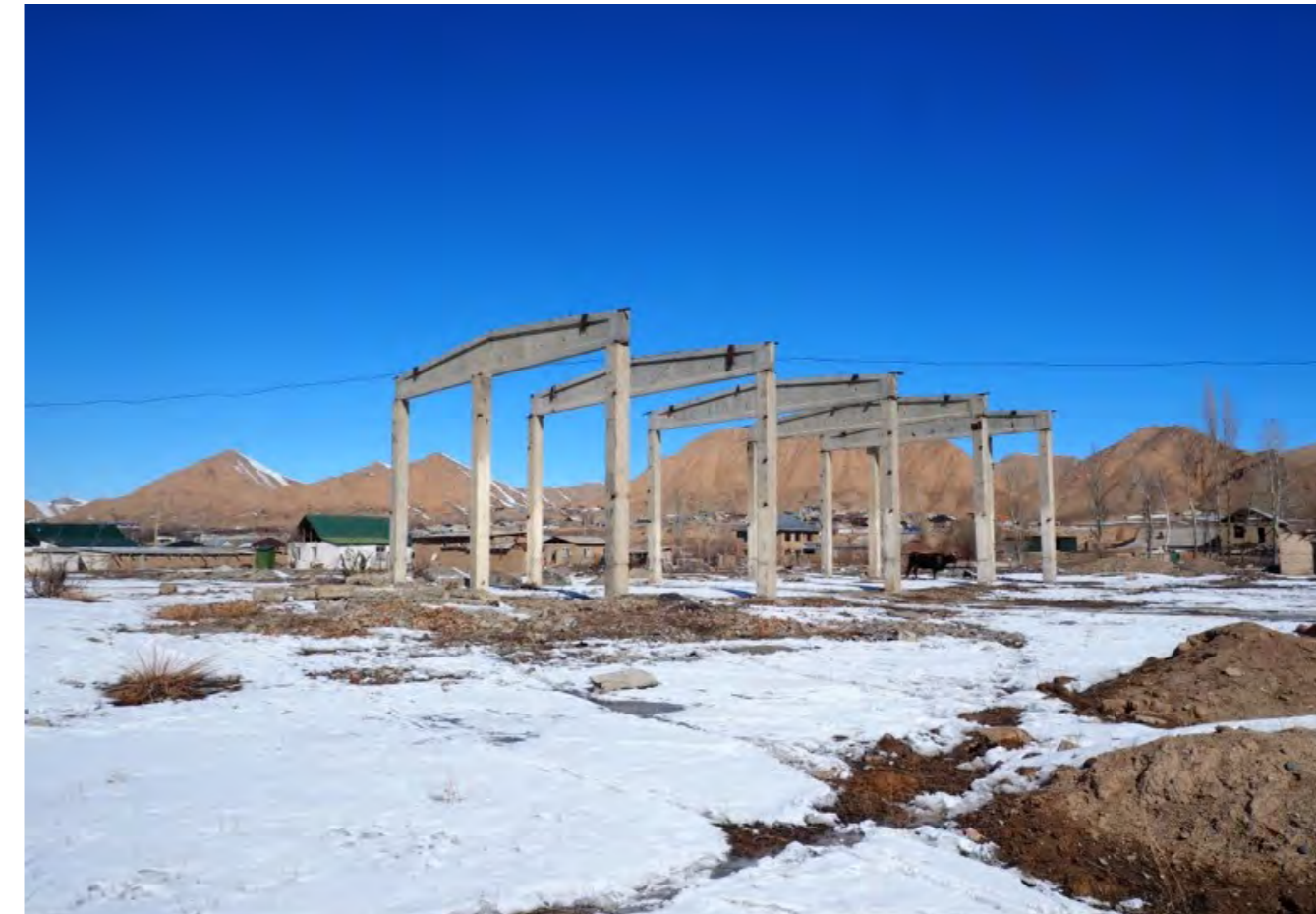
Figure 11. Existing condition of industrial structures
