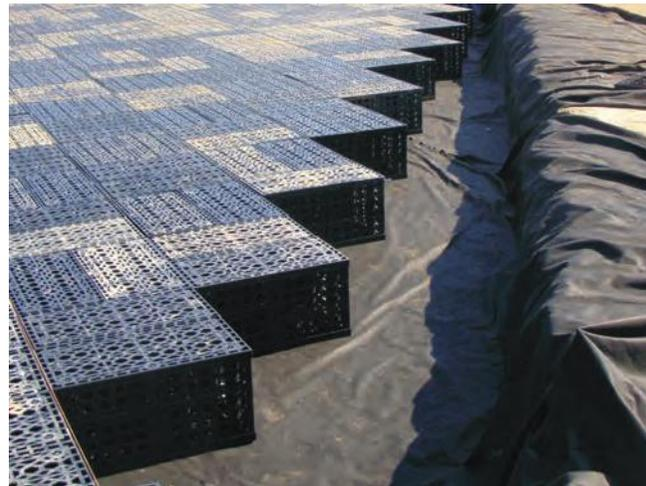
Figure 92. Modular stormwater retention tanks
