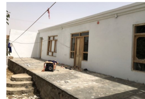
HOUSING AFTER REPAIRS
