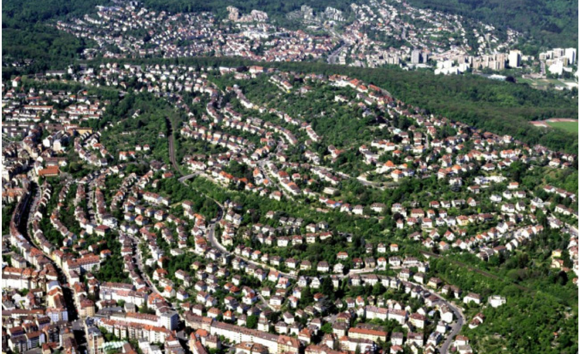
Fig 8. View of ventilation corridors in the city of Stuttgart, Germany
