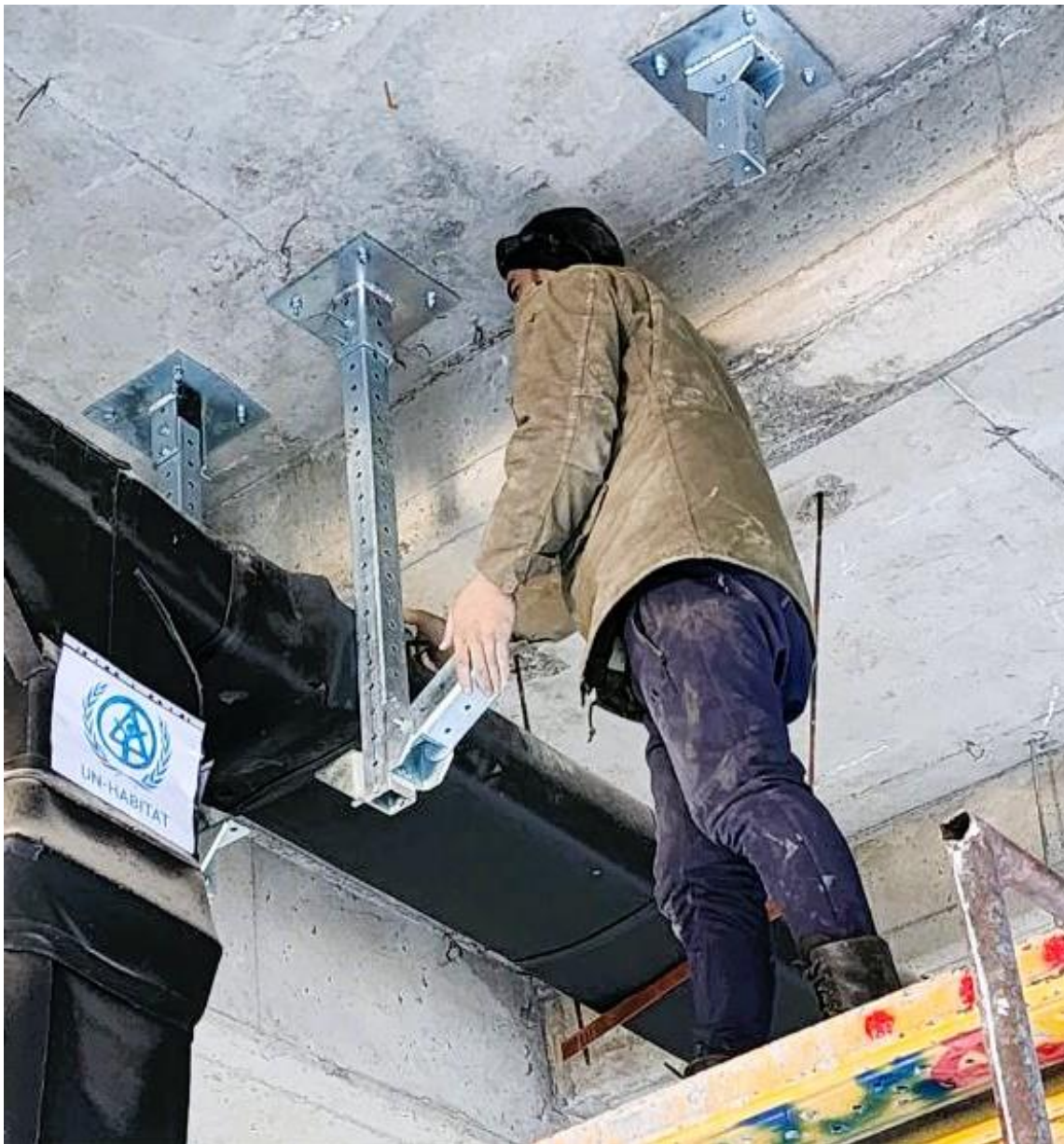
Retrofitting of Piping System, A. Tabarsi Hospital, Sari
