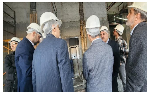
Sari hospital- retrofitting implementation
