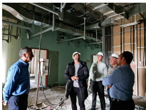
Boushehr hospital- retrofitting implementation
