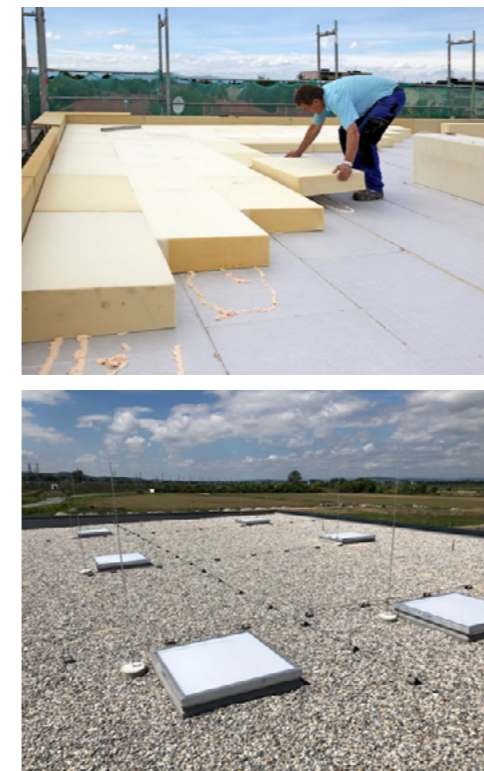
FIGURE 3-13 EPS / XPS / PU sheets in use as insulation for flat roofs 43
