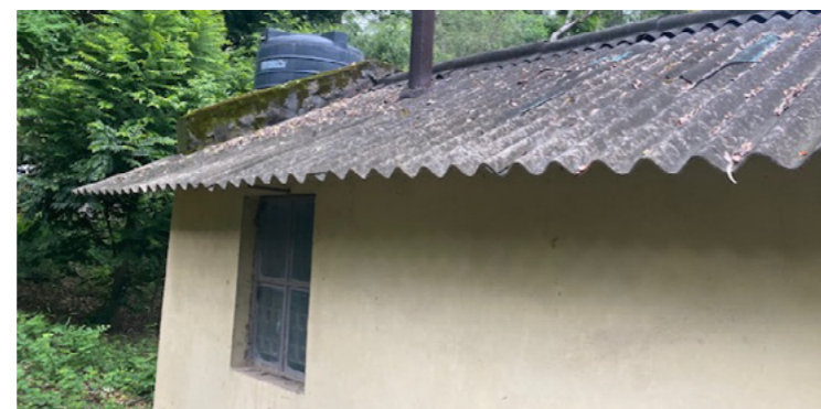
FIGURE 3-12 Corrugated Asbestos Sheets in use (photo credits: Arne Ragossnig)
