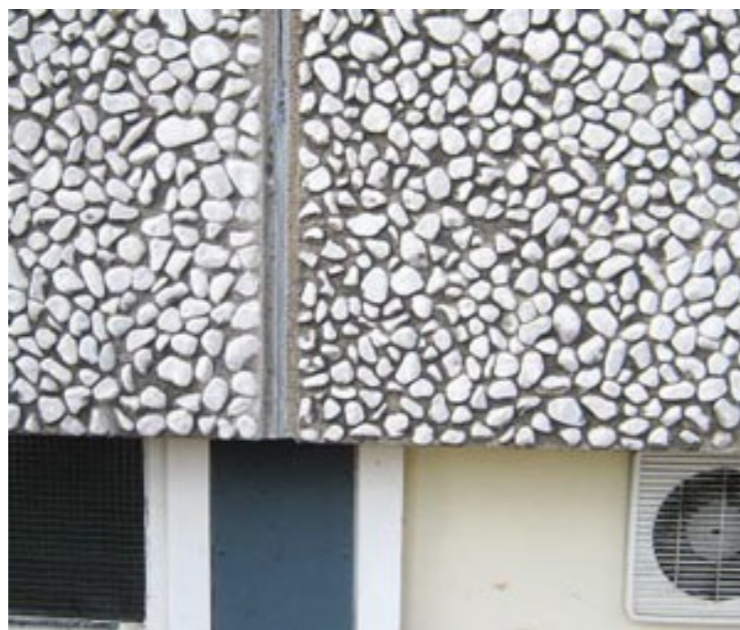
FIGURE 3-17 Expansion joints in use 46
