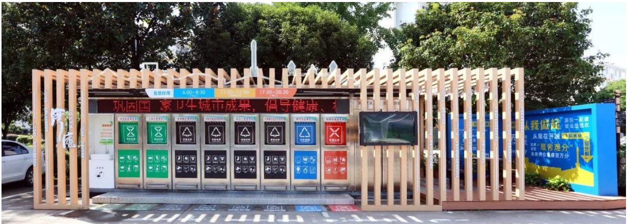
Figure 3-4 Carbon Neutral Hut for Waste Sorting in Wandu Village © LIU Xiao
