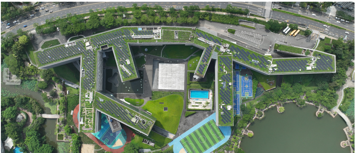
Figure 4-7 Bird's eye view of Vanke Center © Vanke Foundation
