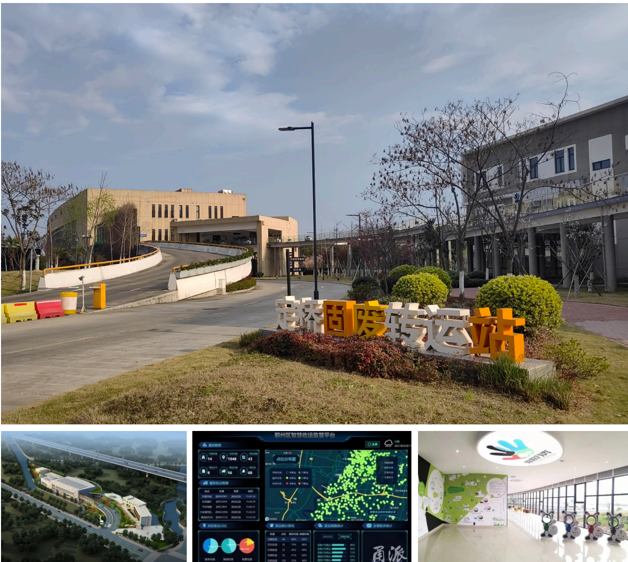
Figure 3-8 Yinzhou District MSW Sorting Transfer Station (Dingqiao Solid Waste Transfer Station) © LIU Xia
