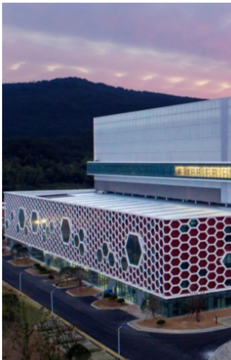
Figure 3-9 Haishu District MSW Incineration Plant © SUS Environment
