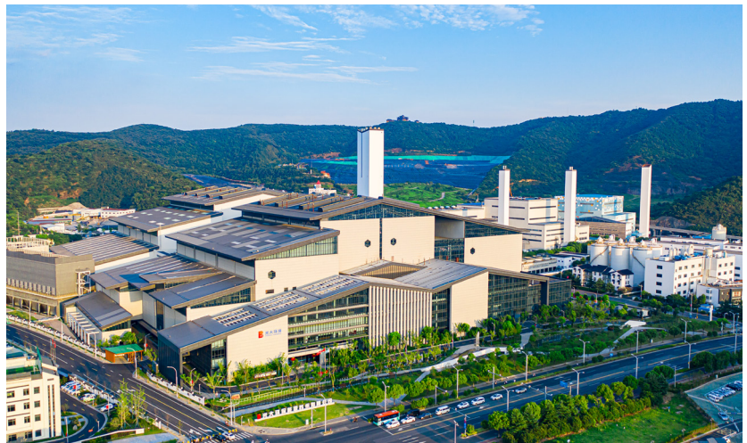
Figure 2-15 Suzhou Qizishan Waste to Energy Plant © Suzhou Environment Sanitation Management Division
