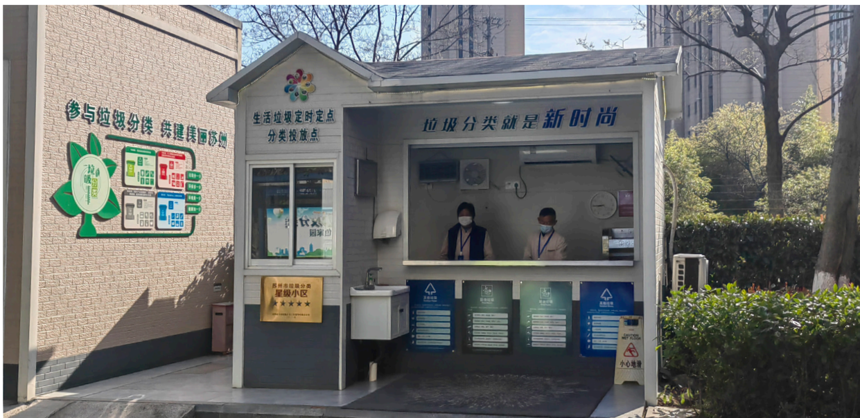
Figure 2-4 Waste collection kiosks in Meisong Phase III Compound © LIU Xiao
