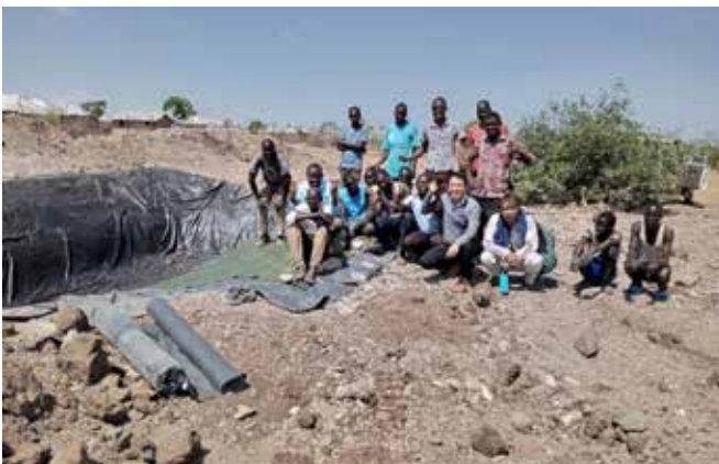
Top left: Construction team including Daiken and local masons. © UN-Habitat
