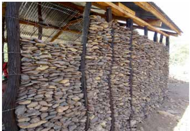
Top left: Exploring dried vegetation housing prototypes; (below) Stone, wire and timber housing prototype built previously in Kalobeyei New Settlement.
