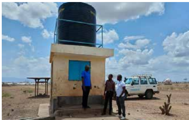
The project team visited the site for the urban livelihoods project at Kang’ura Village. © UN-Habitat
