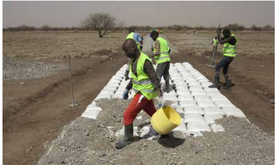
Road construction underway at Kalobeyei New Site. © UN-Habitat
