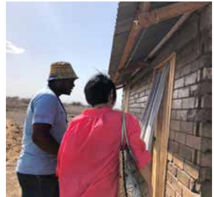
UNIC Director visits Shigeru Ban's durable shelter pilot construction. © UN-Habitat
