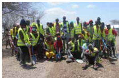
Japanese Do Nou Road construction team. © UN-Habitat
