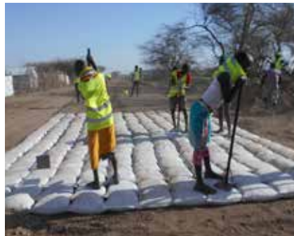
Japanese Do Nou Road construction technology applied to road construction. © UN-Habitat
