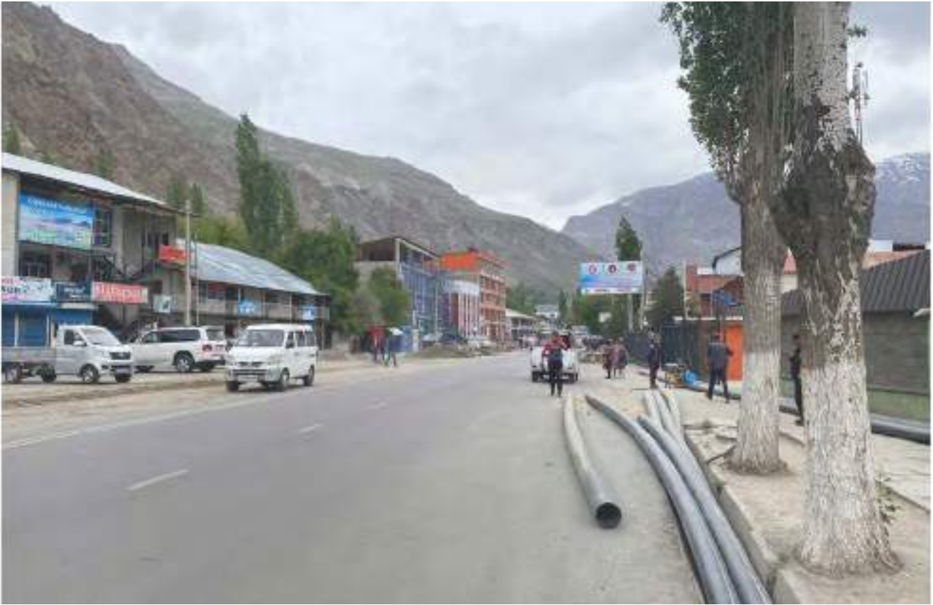
Fig 84. The current state of the main street, UN-Habitat, April 2023
