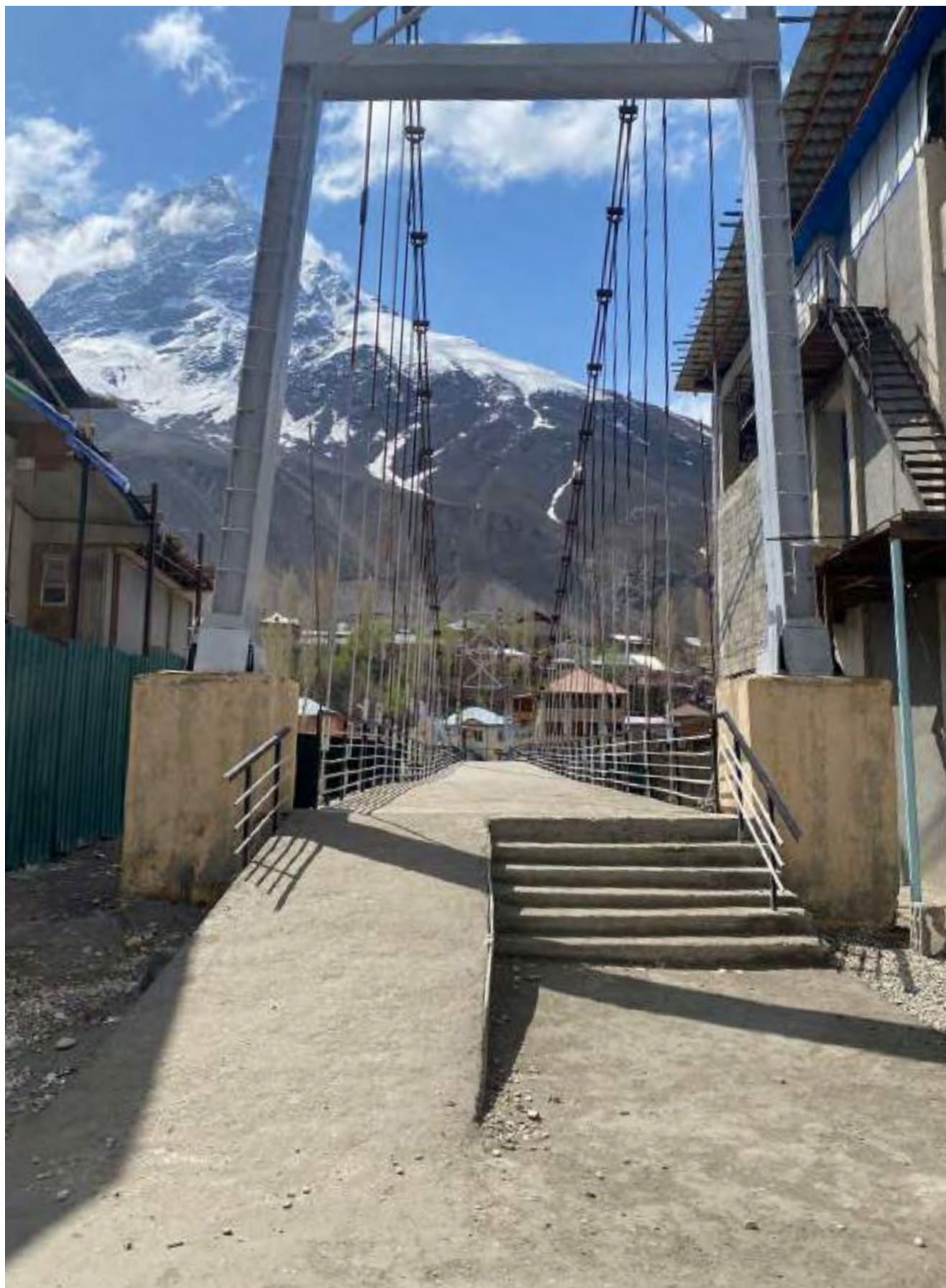
Fig 12. The newly constructed bridge in the market area of Khorog, UN-Habitat, April 2023
