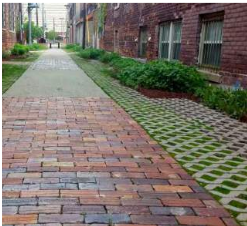
Fig 68. Design of permeable surfaces. Green Alley, Detroit
