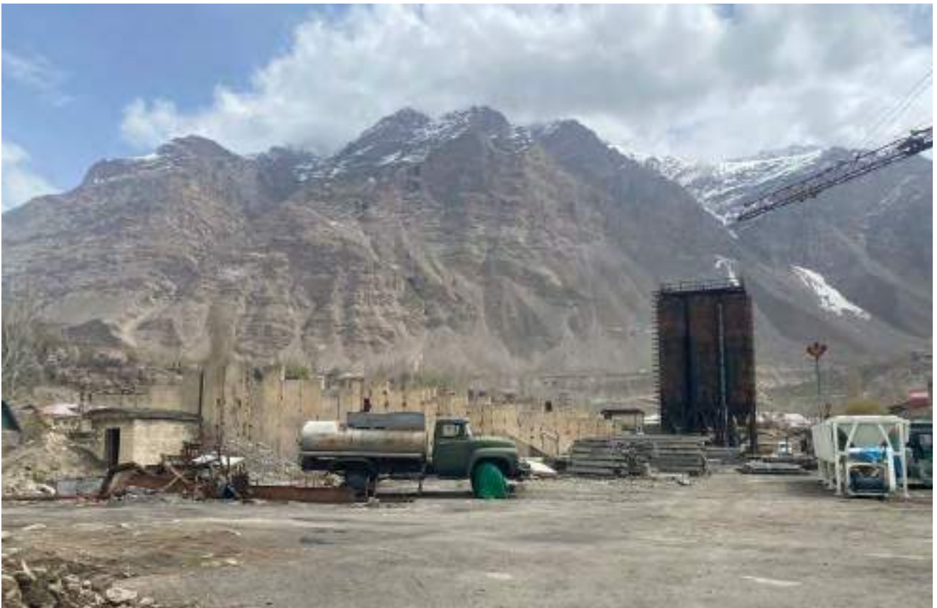
Fig 77. The existing structures of the site B, UN-Habitat, April 2023
