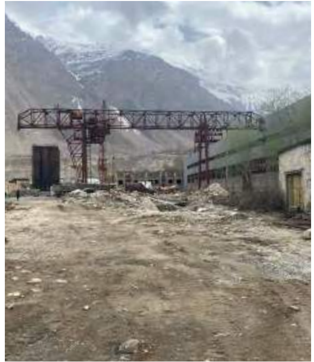
Fig 80. The current state of the project site, UN-Habitat, April 2023
