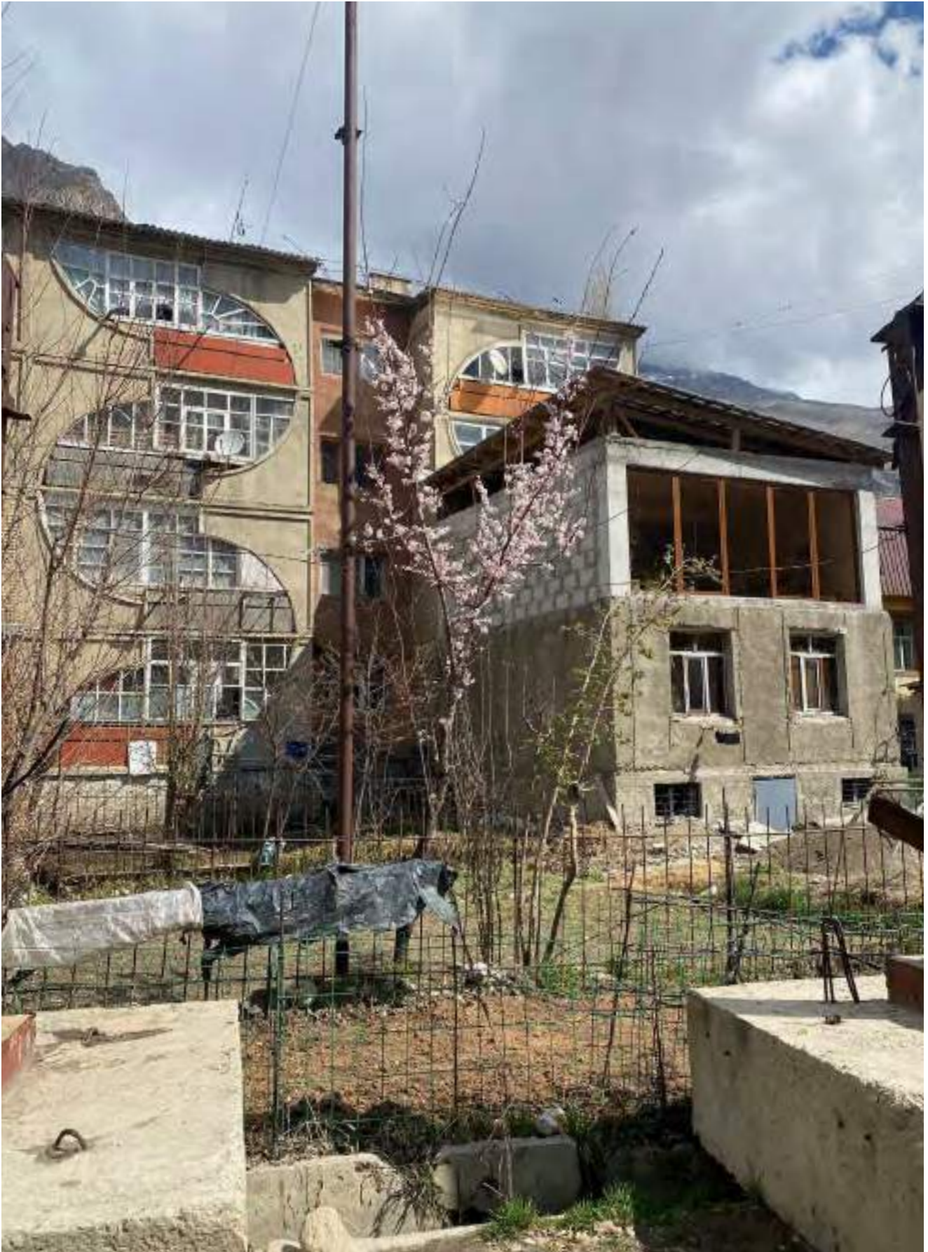
Fig 11. Apartment block in Khorog, UN-Habitat, April 2023
