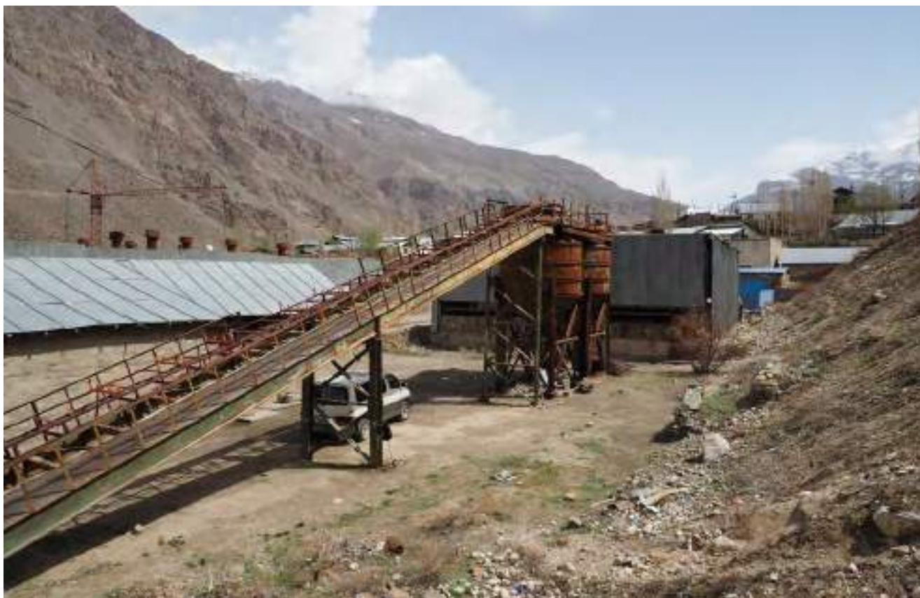
Fig 57. Existing steel ramp, UN-Habitat, April 2023
