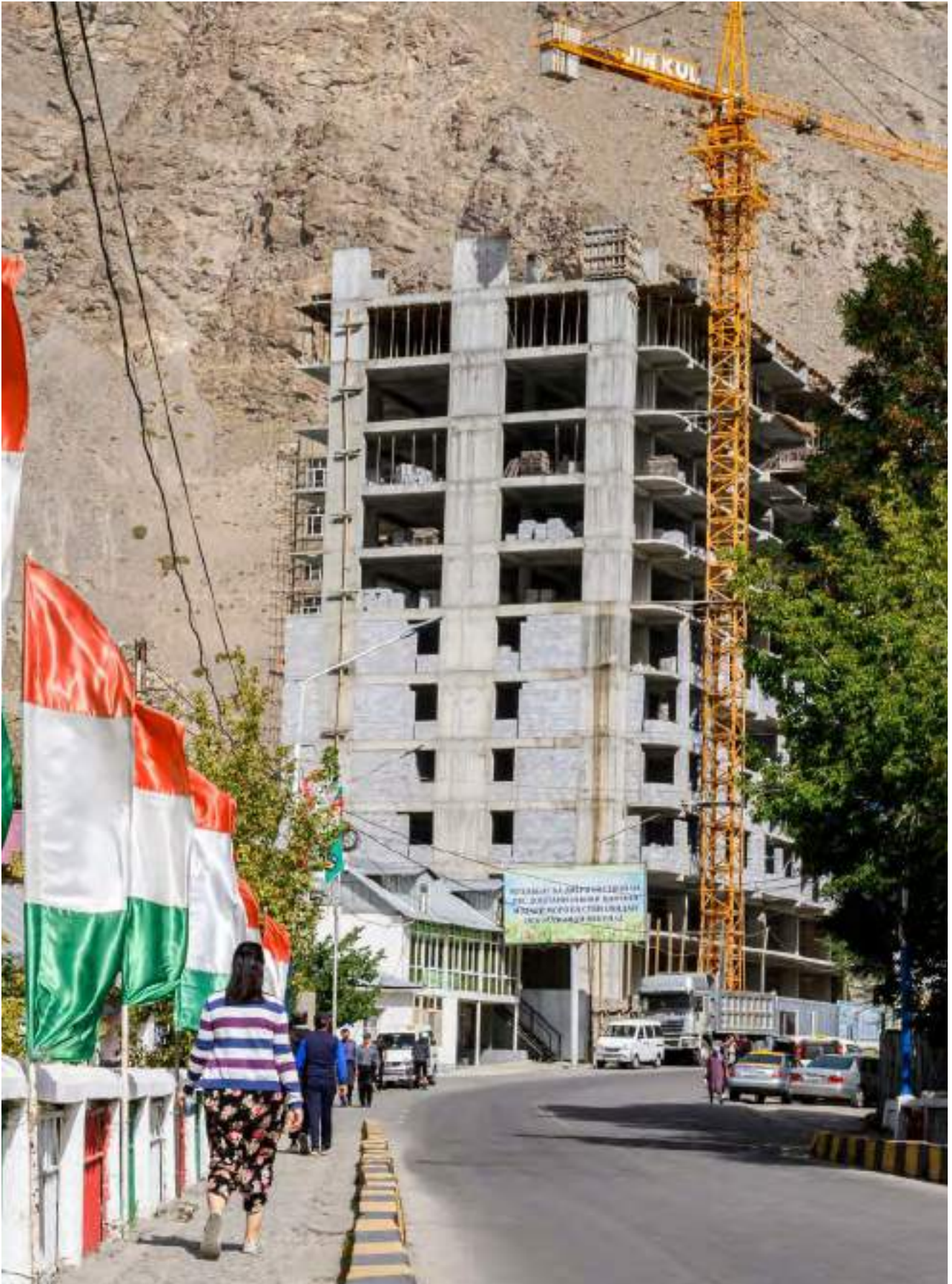
Fig 2. New building being constructed in Khorog, UN-Habitat, September 2022
