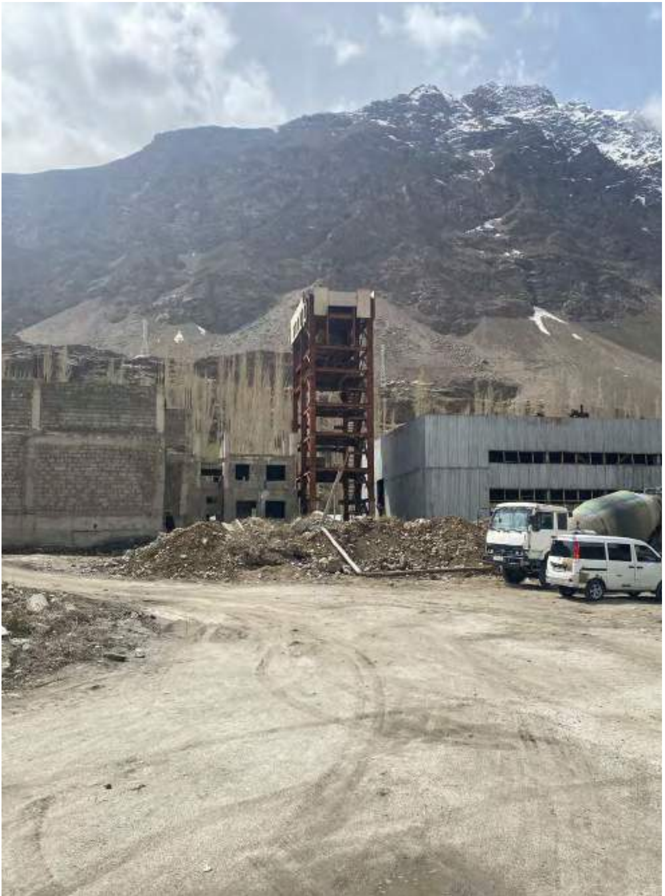
Fig 73. The current condition of the site B, UN-Habitat, April 2023
