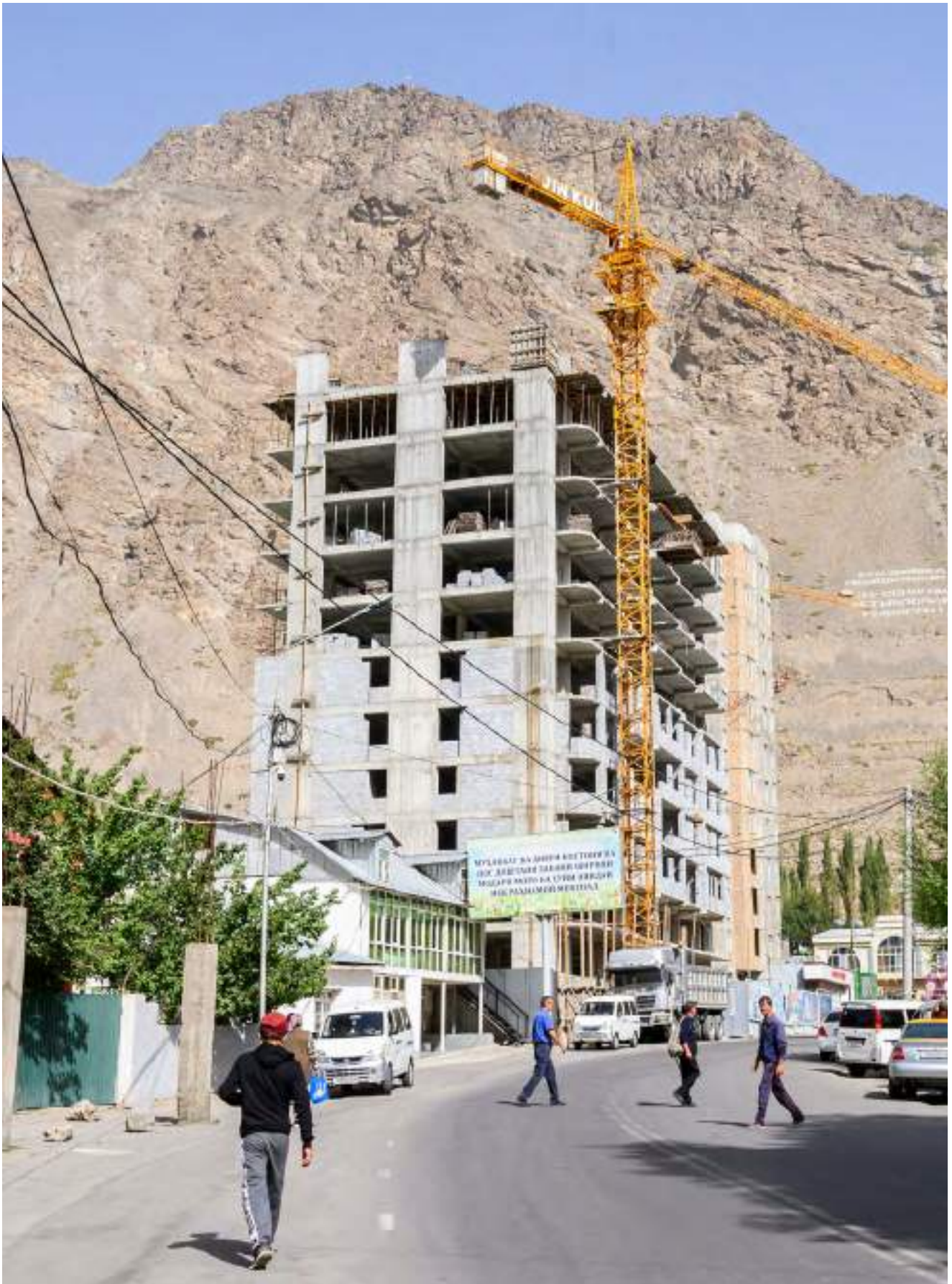
Fig 2. New high-rise building being constructed, UN-Habitat, September 2022
