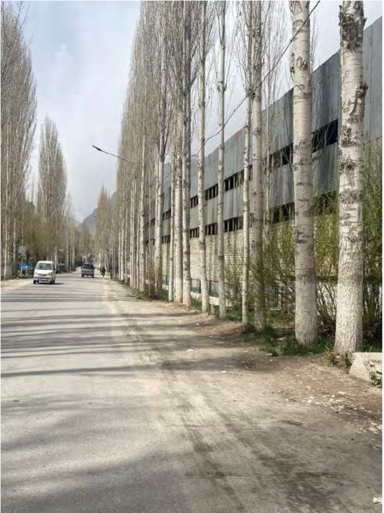
Fig 90. The part of the main street (the loop) adjacent to the site B, UN-Habitat, April 2023
