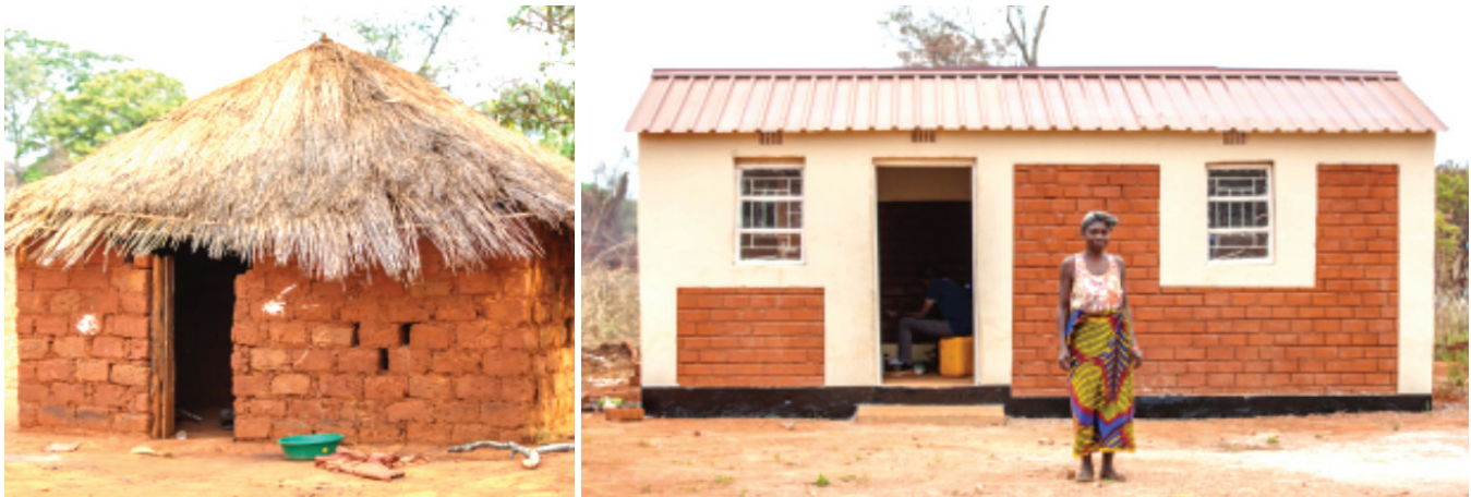
Figure 10 and 11: Before: using traditional soil bricks and thatch roofs. After: ecofriendly low income buildings using SSBs
