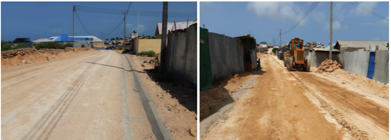
Figure 26 and 27: Constructed a 3km gravel road in Midnimo village (Northern part of Kismayo city); promoting accessibility to the main city for over 8000 people.
