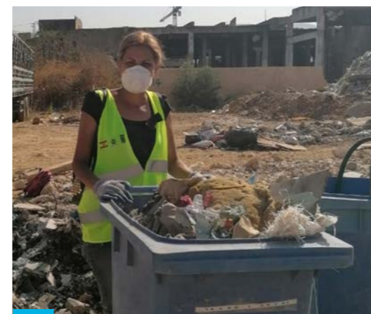
Zeinab Khamis separates the rubble into material type: glass, plastics and metal © UN-Habitat/ Elie Mansour
