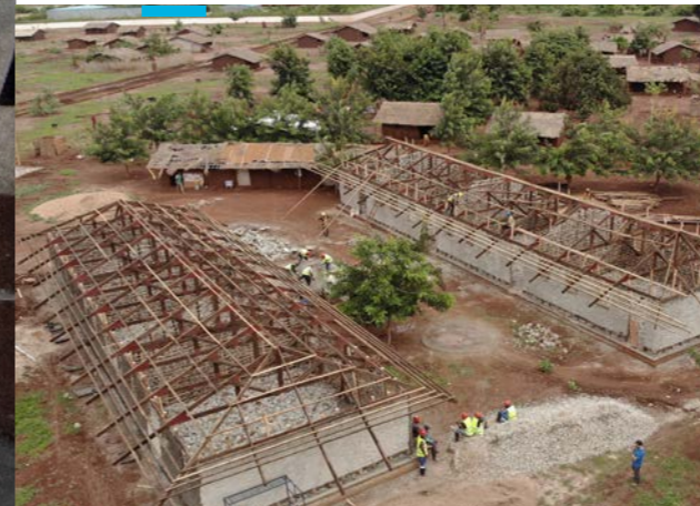
Building mixed material resilient schools with the local communities © UN-Habitat Mozambique
