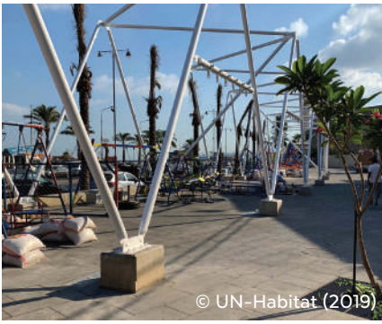
Ongoing Bahr El-Eid public space project
