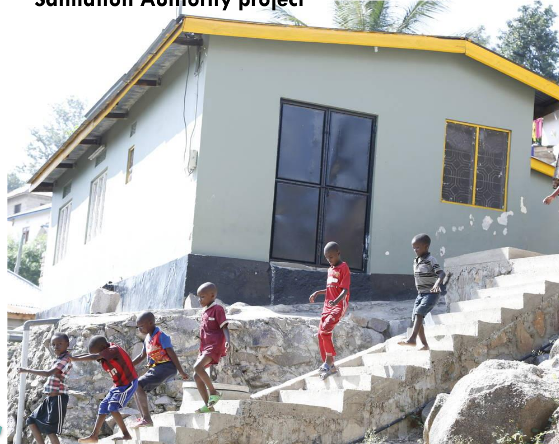
EIB funded Mwanza Urban Water Supply and Sanitation Authority project
