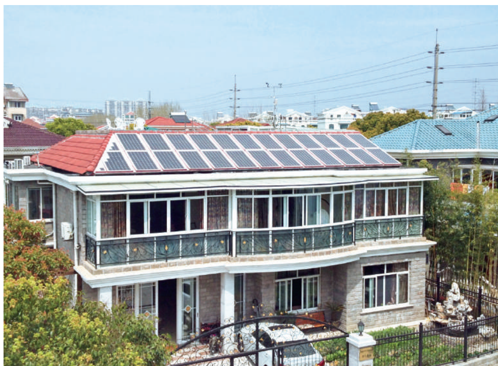
Figure 4.13 Solar Photovoltaic Panels on the Roof of Dwellings of Chongming Island
