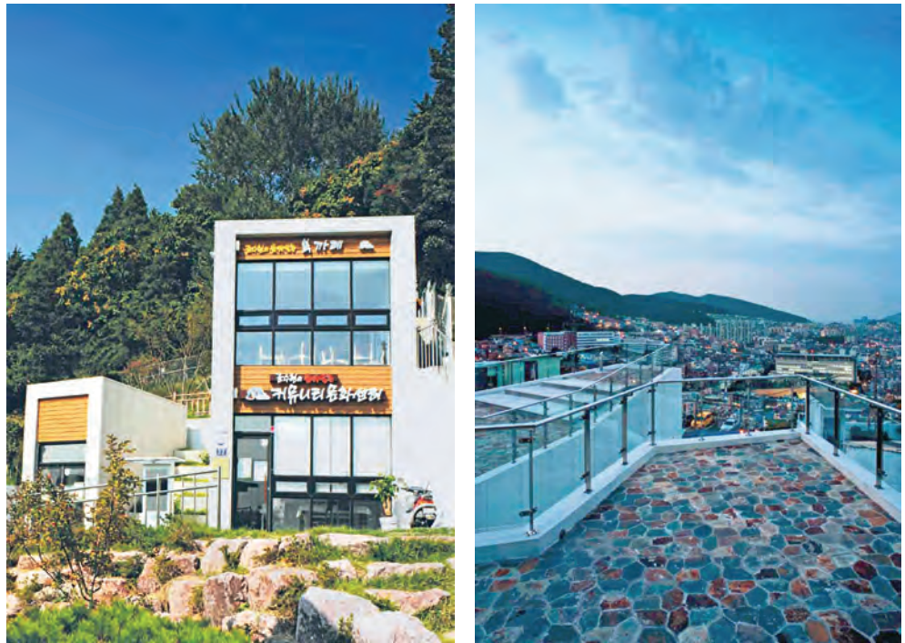
Figure 3.22 Recently Constructed Cultural Facilities in the Sanbokdoro Region
