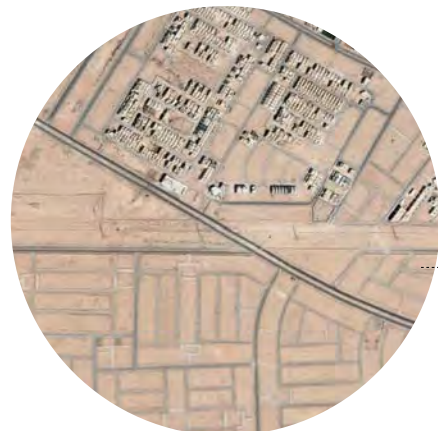
3. Emerging residential development and infrastructure
